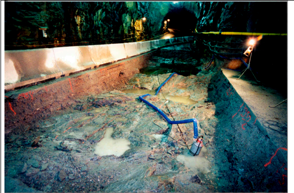
Appendix 8A. Photos showing the pit-floor in the TBM assembly hall (photos: Lars Andersson, SKB). Overview of the pit looking up the ramp
