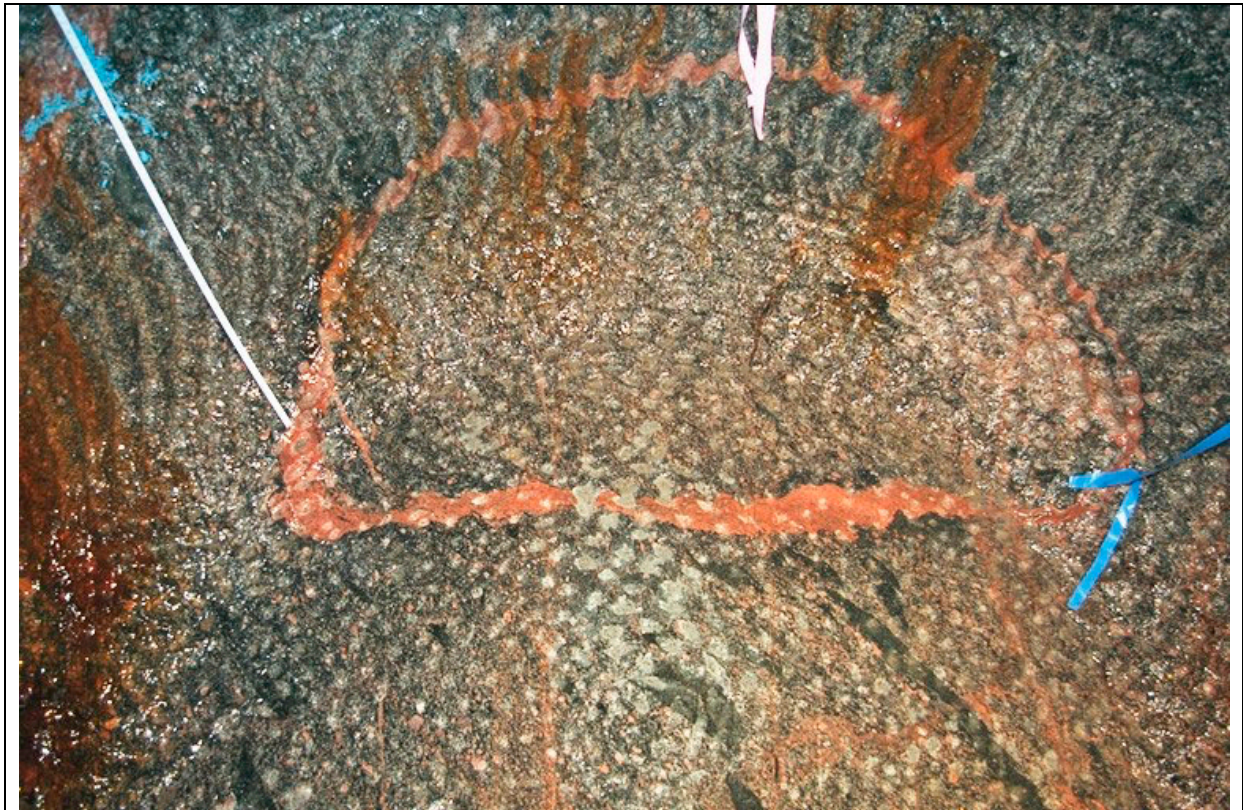
Appendix 11E. Photos from deposition hole DA3147G01 (photos: Lars Andersson, SKB). Bottom part of the hole. Rock types: Äspö diorite (greyish) with minor greenstone xenoliths (dark grey – black) and fine-grained granite (pinkish red). Water bearing fracture with rust staining below. The grooves are a result from the drilling. The white, pink and blue ribbons were used during the mapping procedure not only for orientation but were also a part of a grid system
