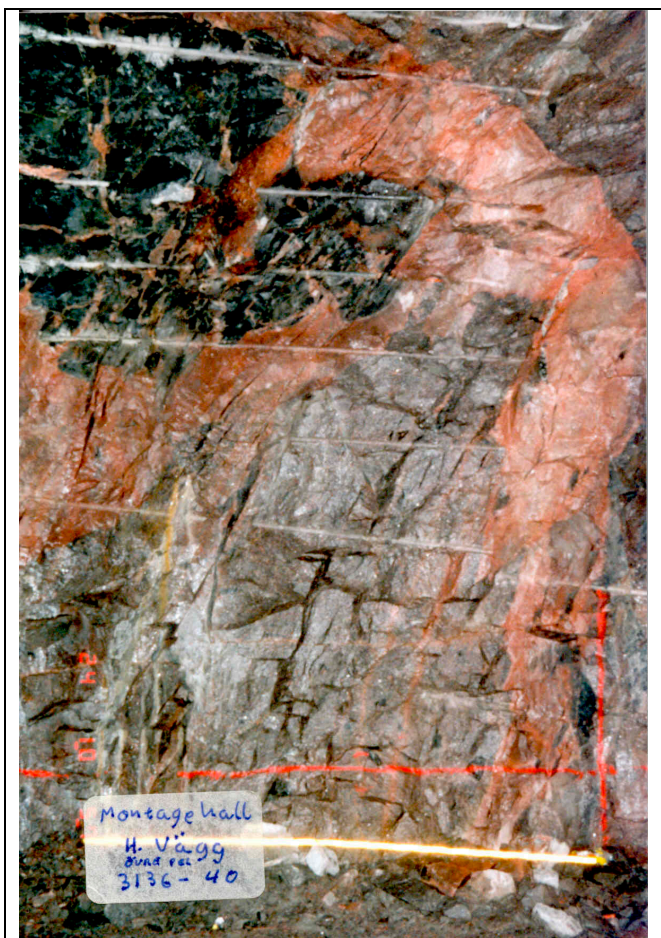
Appendix 3D. Photos showing the interior of the TBM assembly hall (photos: Geologist team at the time, SKB). Right side wall, section 3/136-3/140. Mainly Äspö diorite (grey) with fine-grained granite (brownish red). A greenstone xenolith (black) is seen in the left upper corner of the picture
