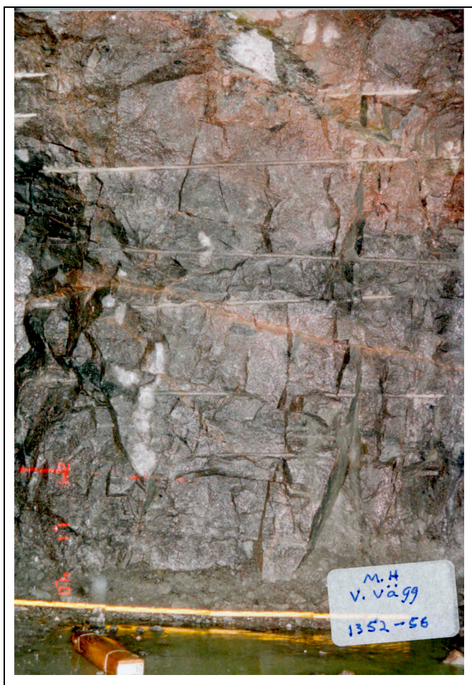
Appendix 3B. Photos showing the interior of the TBM assembly hall (photos: Geologist team at the time, SKB). Left side wall, section 3/152-3/156. Mainly Åspö diorite (grey) and fracture with some oxidation (reddish brown)
