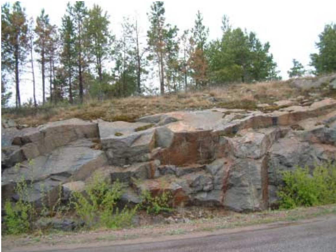
Figure 3-1. Examples of joint character and orientation in local exposures.
