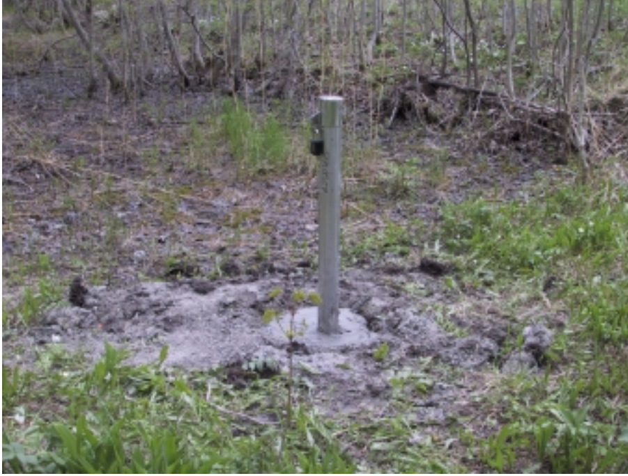
Figure 4-2. Groundwater monitoring well SFM0027. Cover pipe in stainless steel for protection of the HDPE stand pipe.
