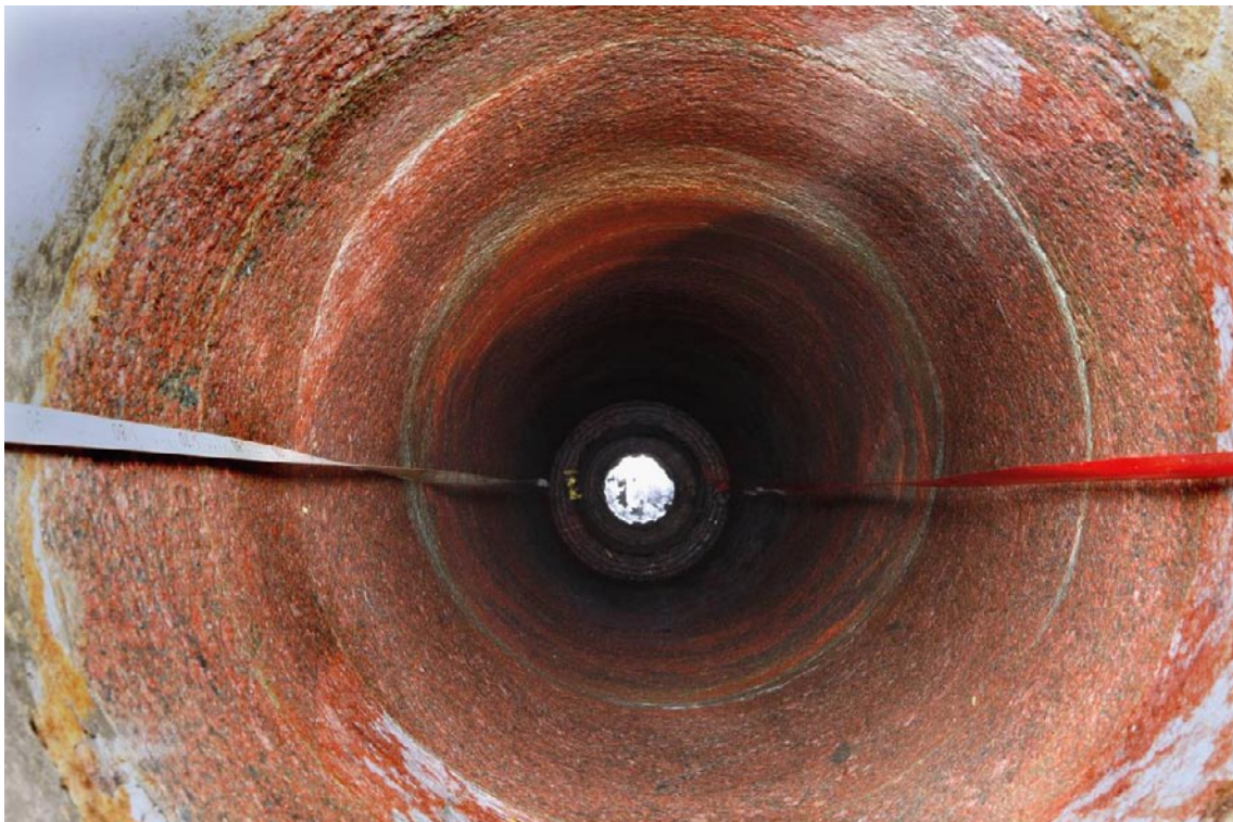
Figure T-8. Photograph of borehole KQ0048G05 in Field Test 3 before initiating the heating phase.
