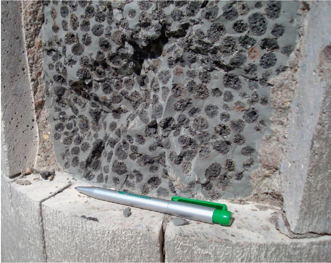
Figure 7-7. Photograph from sealing test in 50 mm pellet filled slot. The voids are completely filled and the contact surface is tight (Photo R Glamheden).
