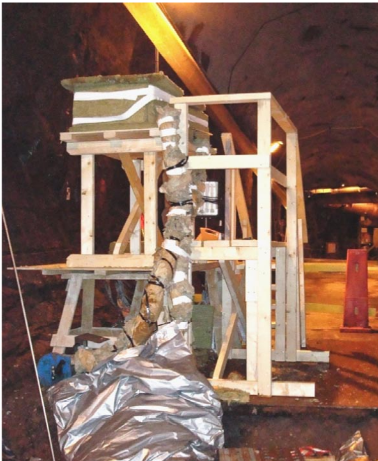
Figure 3-6. Shows the tank and part of the pipe work of the wetting system installed in the last field test. Both the tank and the pipes were well insulated to minimize heat loss from the system (Photo C-R Lindqvist).
