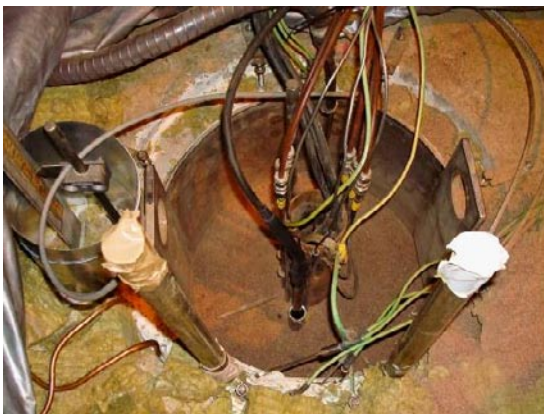
Figure V-13. Shows KQ0046G04 after replacement of a heater element in Field Test 4.
