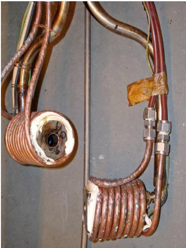
Figure U-7. Shows the state of the monitoring camera after completion of Field Test 1.
