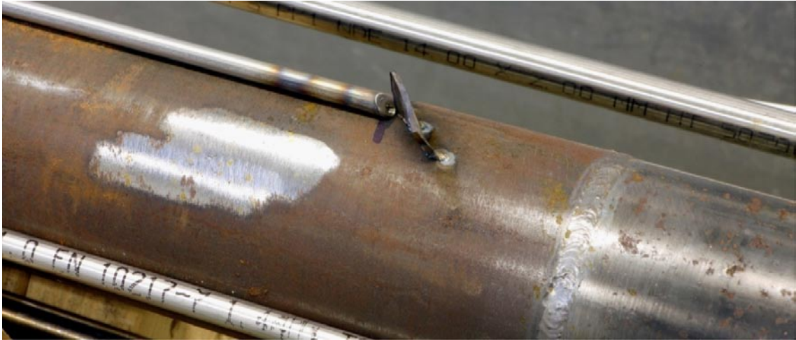
Figure 3-5. Close-up view of the pipe and the drip plate included in the wetting system used in the second heating test (Photo C-R Lindqvist).
