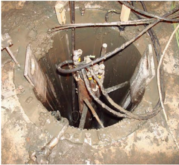
Figure V-14. Shows the equipment and the pellet filled slot before en after the grouting of the pellet filled slot in KQ0046G03.
