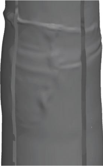
Figure S-1. Laser scanned mesh of heating hole KQ0046G04. Spalling can be seen as a vertical trace along the mesh, at a location between ca -446.3 and -446.75 m.
