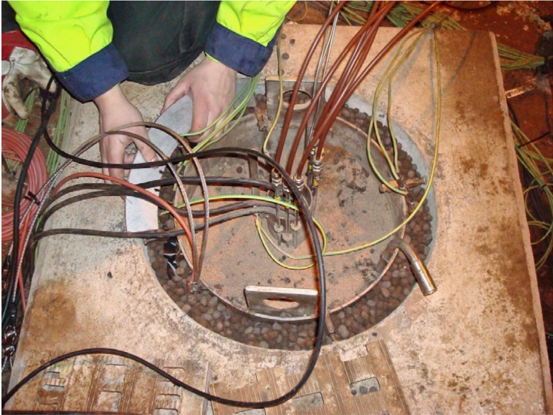
Figure 3-2. Photograph of the pellet filled slot during preparation of Field Test 4 (Photo R Glamheden).
