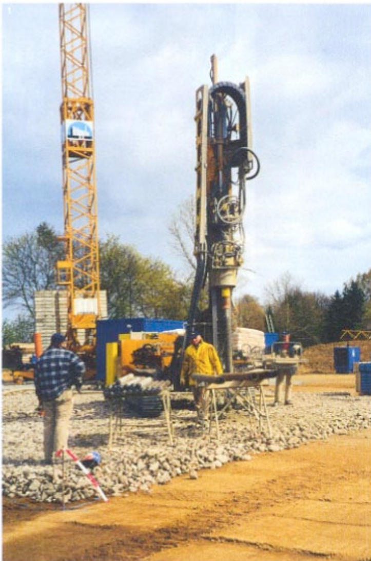
Figure 5-10. Grouting from surface, before sink shaft excavation /Ahlbrecht 2005/.
