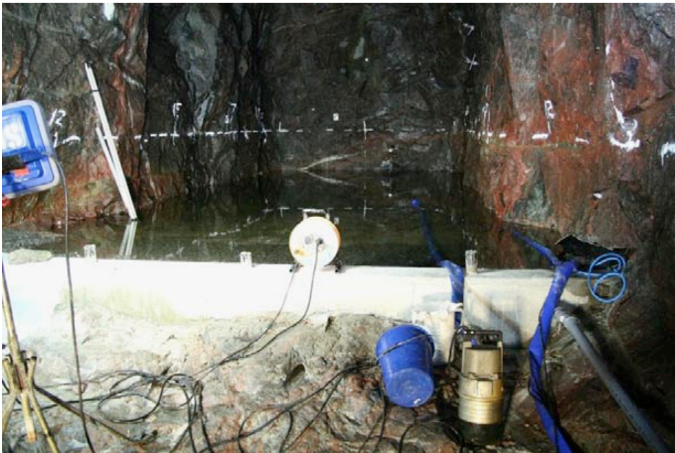
Figure 5-8. Measuring the inflow in measuring weirs, photo from SKB:s sealing project at great depth /Funehag 2008/.
