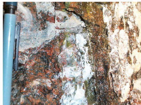
Photo 7: Structure2198m at 2198B (Site 3) The structure comprises of several fault planes lying in a thin zone of moderate mylonite (centre) between weak mylonite (right) and undeformed diorite (left). White material is re-precipitated grout. Width of photo ca.15cm.
