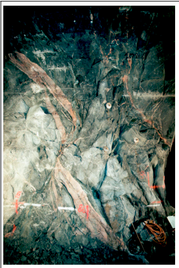
Appendix 3B. Photos showing the tunnel interior. Part of the tunnel wall, right hand side, section 84-88. Dislocated fine-grained granite (reddish) in Äspö diorite and greenstone (both grey). Photo: Lars Andersson, SKB.
