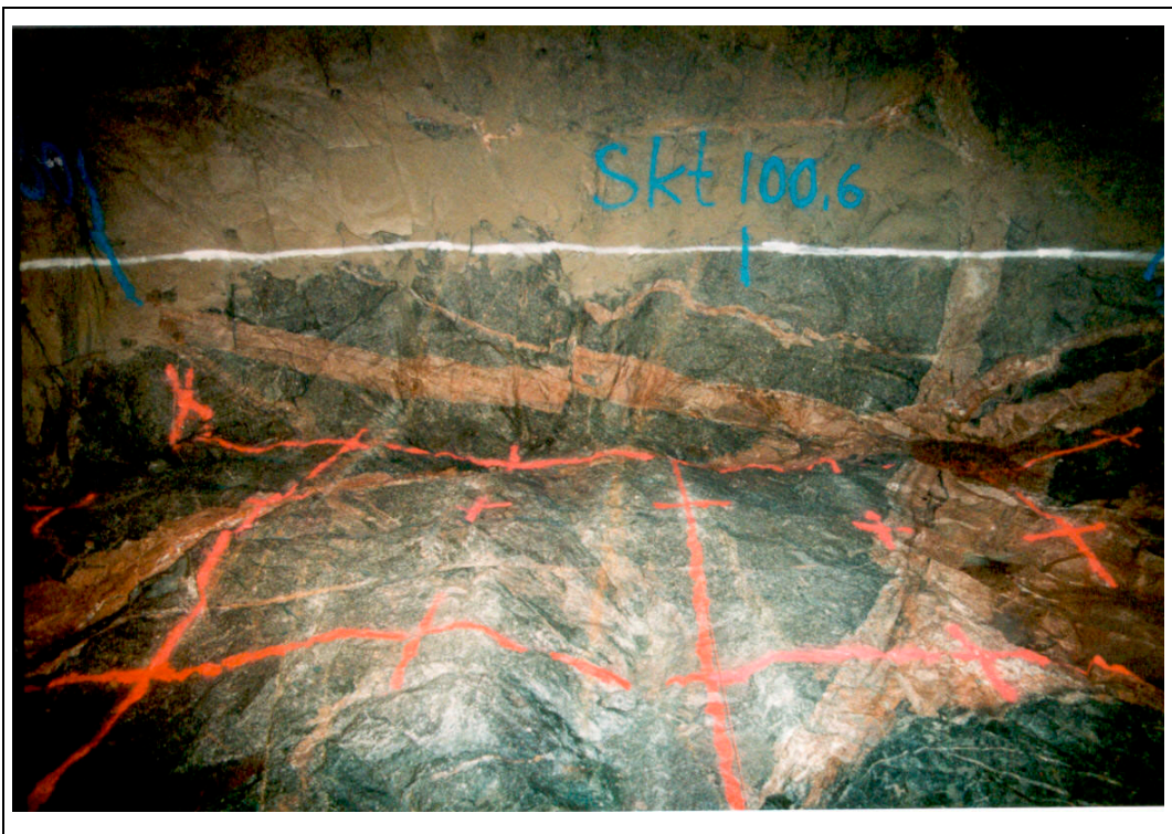
Appendix 3D. Photos showing the tunnel interior. Part of the tunnel floor and front with intersecting fine-grained granite dykes (reddish) in Åspö diorite (grey). One of the fine-grained granites in the front has been dislocated. Photo: Lars Andersson, SKB.
