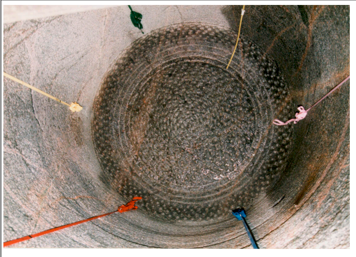
Appendix 14C. Photos from deposition hole DD0092G01. Bottom of the deposition hole composed of Åspö diorite. Photo: Lars Andersson, SKB.
