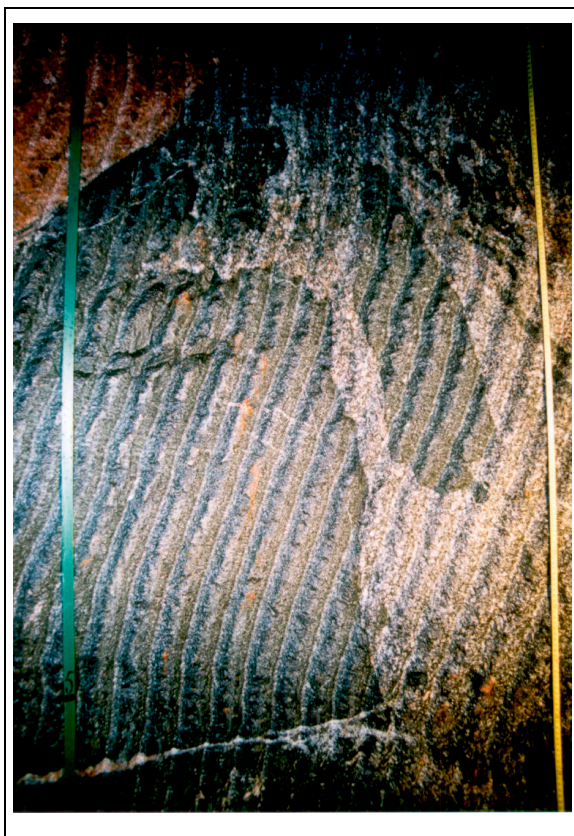
Appendix 10B. Photos from deposition hole DD0086G01. Part of the hole, section 4-5m, showing some rock types: Äspö diorite (grey), greenstone (black-dark grey) and fine-grained granite (reddish) and the grooves resulting from the drilling of the hole. Photo: Lars Andersson, SKB.
