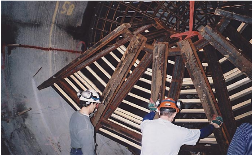
Figure 5-8. Reassembling the formwork at the location of the plug.
