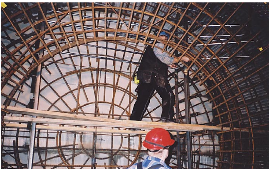
Figure 5-5. Installation of the cooling pipes within the reinforcement cage.
