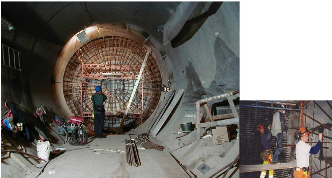
Figure 5-4. Installation of reinforcement.
