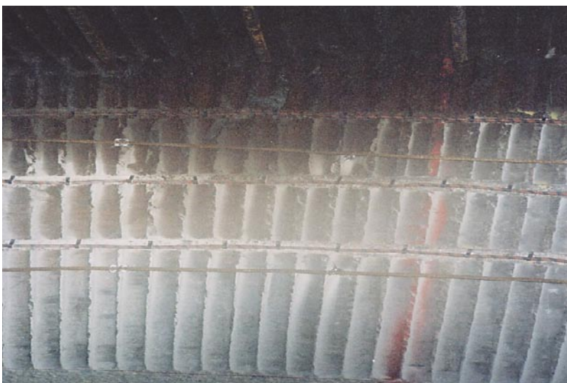
Figure 5-3. Three notches were cut to fit the grouting tubes.
