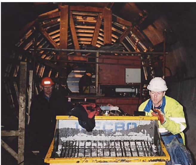
Figure 5 -11. Assembling and testing of the concrete pump.
