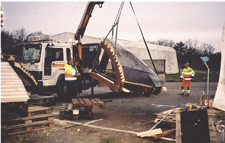
Figure 5-7. Loading of formwork parts for transportation down the tunnel.
