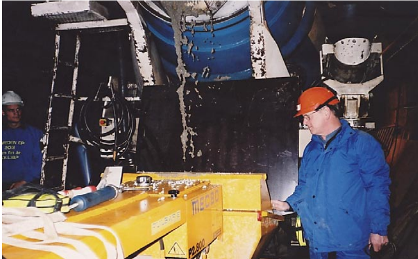
Figure 5-12. The fresh concrete viscosity condition was continuously checked.
