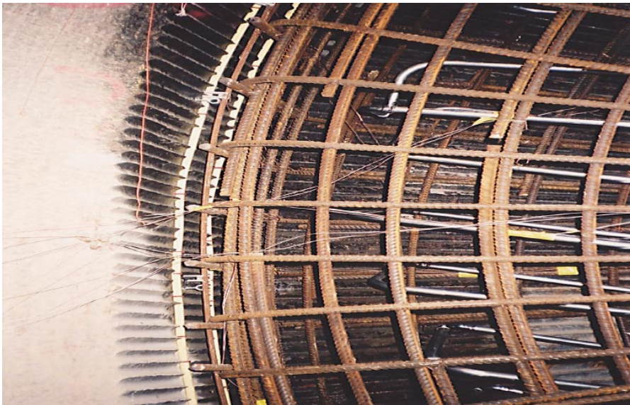
Figure 5-6. Monitoring instruments and cooling pipes are installed within the reinforcement cage.
