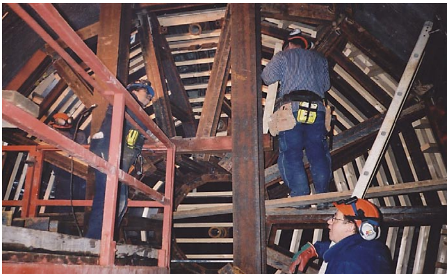
Figure 5-9. Two vertical beams were installed as struts to support the formwork.
