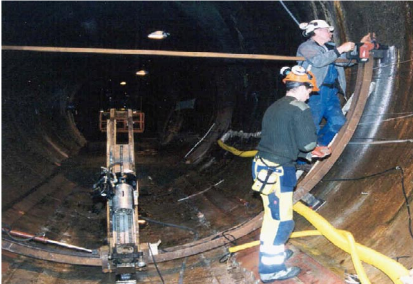
Figure 4-4. Installation of the rig to the rock wall.
