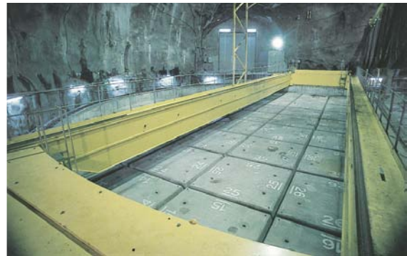
View over top of silo
