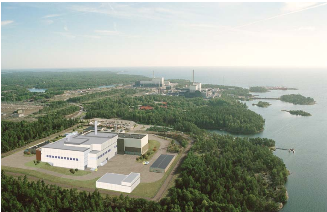
Figure 2-8. Encapsulation plant for spent nuclear fuel integrated with Clab.
