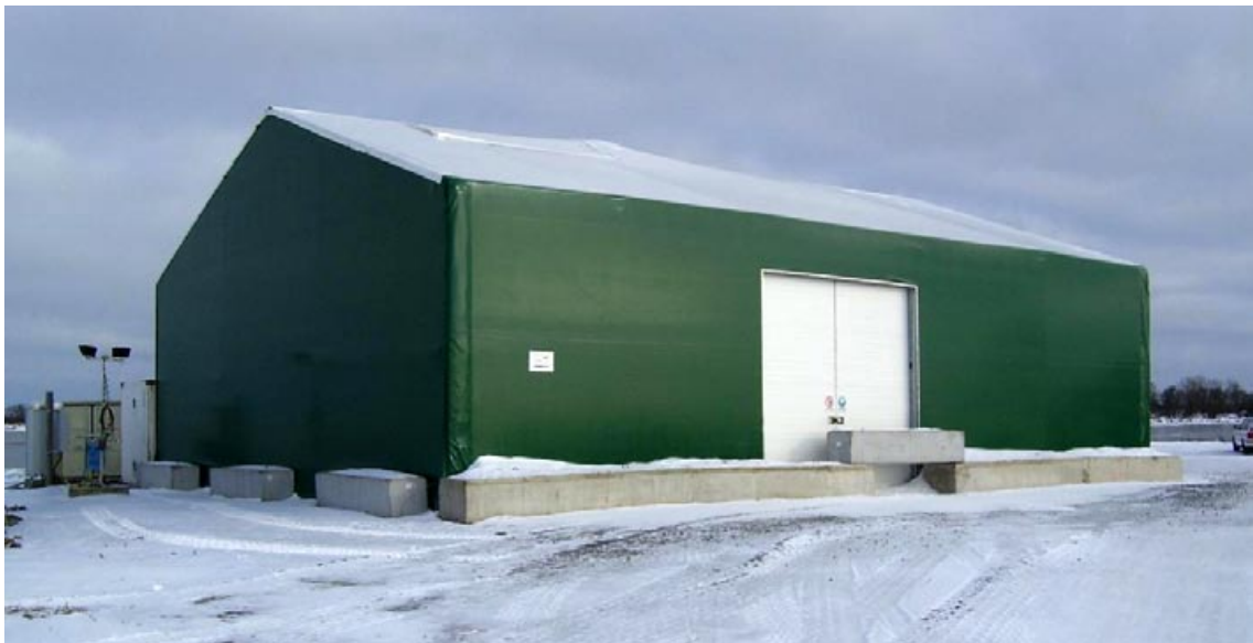
Figure 5-1. Drill site DS102 with borehole KFR102A, located farthest east on the pier at Asphällskulten. To protect the water system and other sensitive equipment from freezing, a tent with electrical heaters was used to keep the temperature above zero. Another advantage with the tent was improvement of the working environment.
