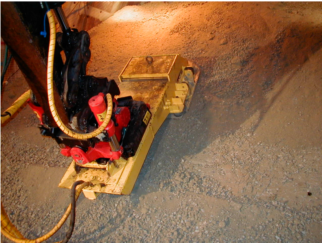
Figure 5-6. The slope compactor.
