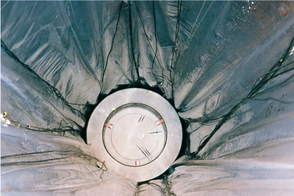
Figure 4-3 A photo taken after installation of the bottom block and the first bentonite ring, showing also the plastic sheet and several transducers installed in the bottom block.
