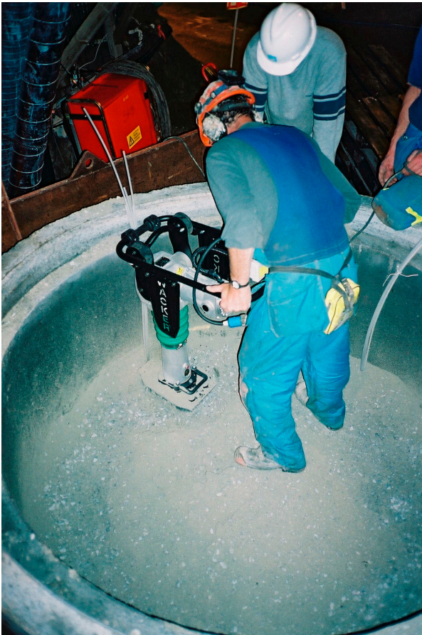
Figure 5-13. Test compaction for the deposition holes.
