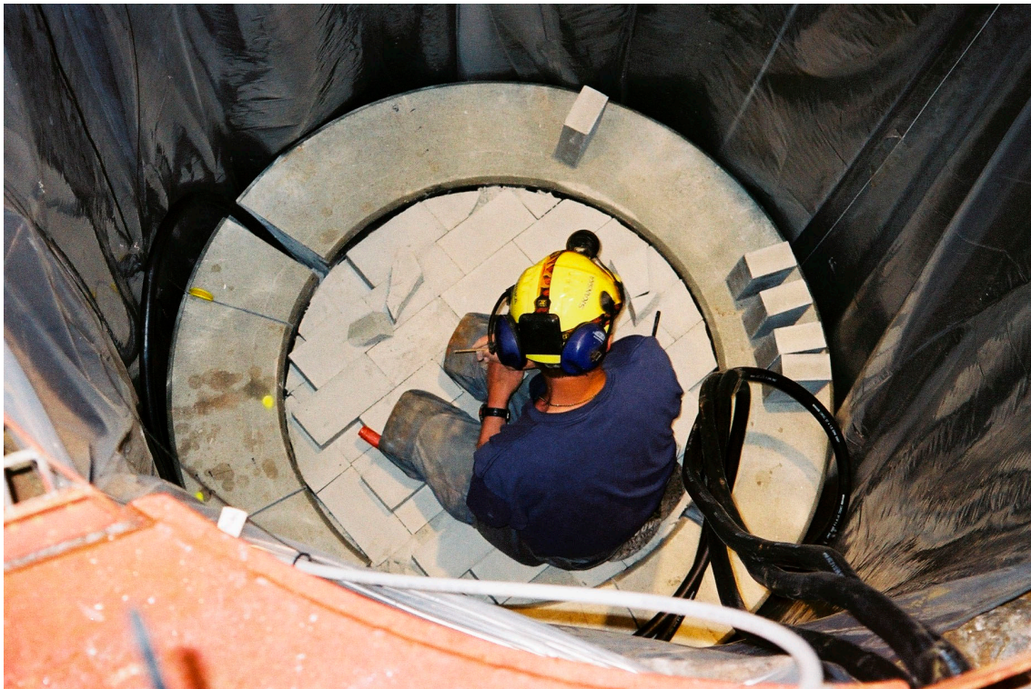
Figure 4-8 Bricks of bentonite placed on top of the lid of the cansiter.
