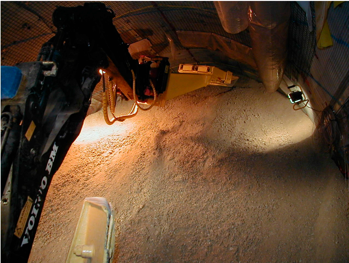
Figure 5-5. The roof compactor.
