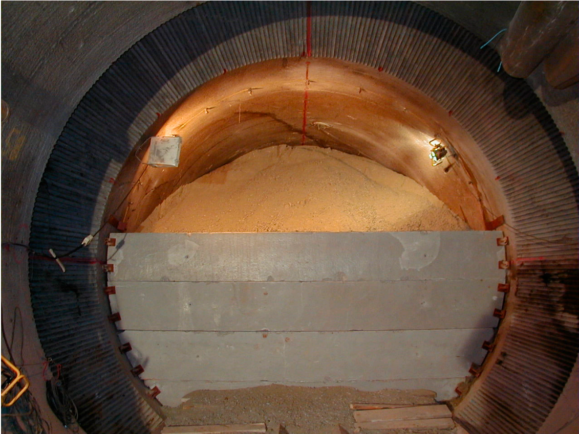
Figure 5-14. Installation of the concrete beams for the retaining wall.
