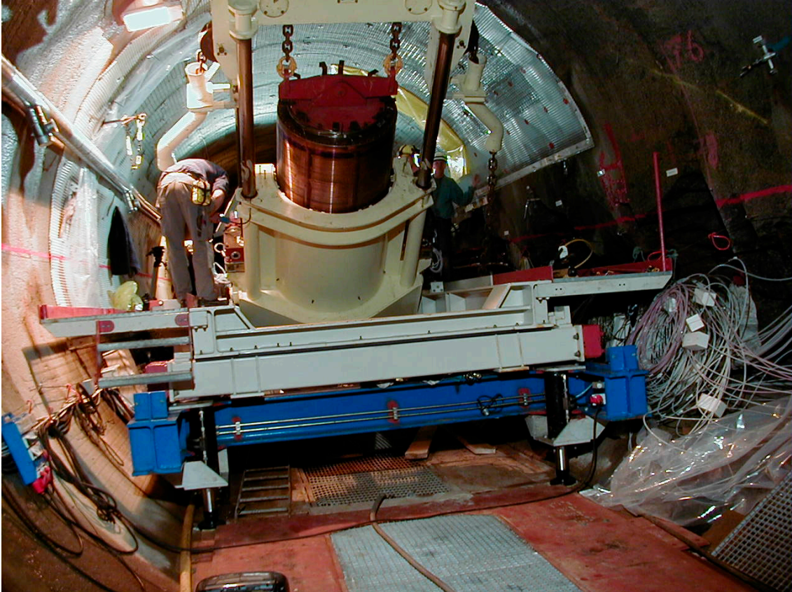
Figure 4-5 The canister tilted into the deposition hole.
