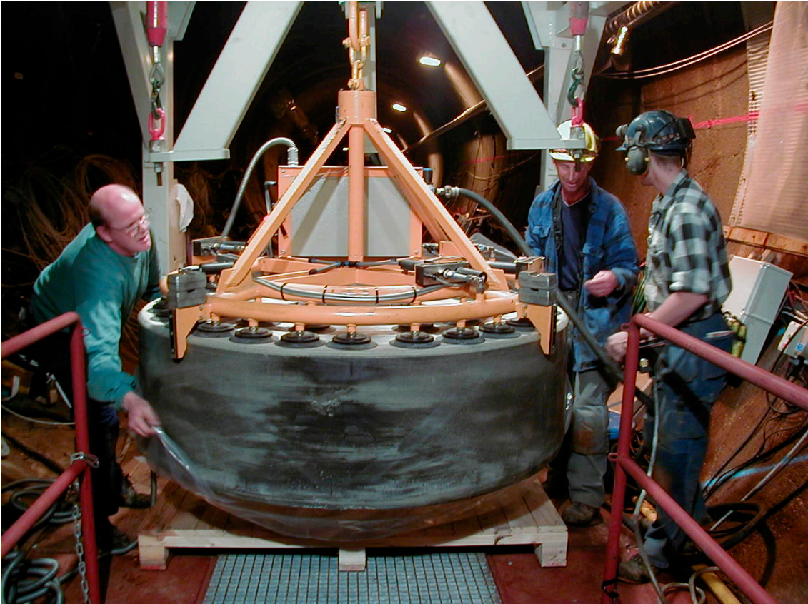
Figure 4-10 A bentonite block hoisted from the deposition hole, placed on a pallet and wrapped in plastic.
