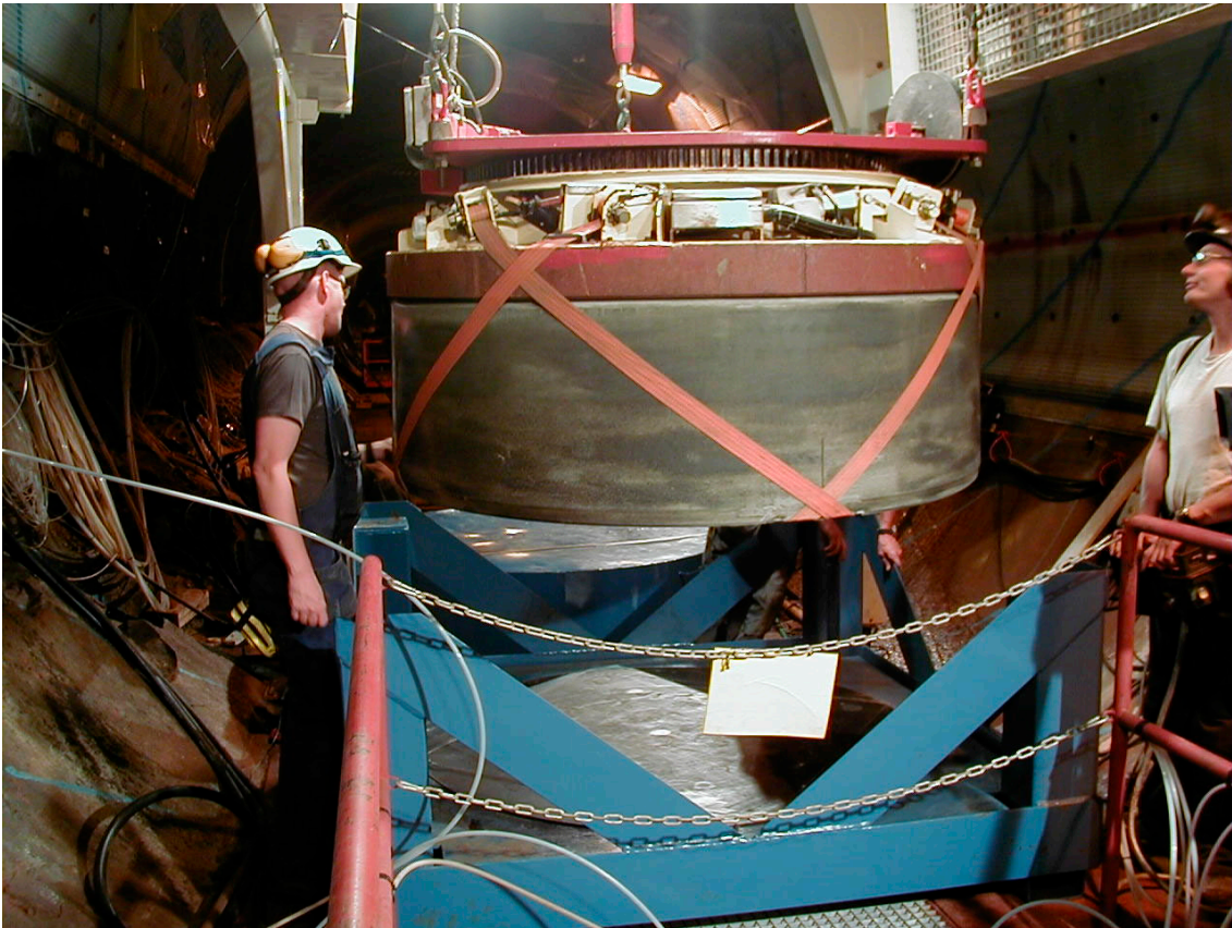
Figure 4-2 A bentonite block attached to the lifting equipment with four straps.
