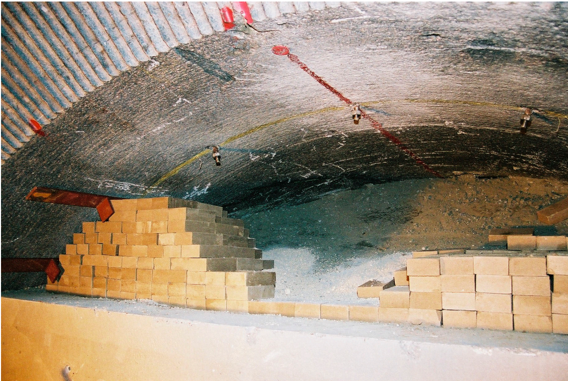
Figure 5-15. Placing blocks and pellets in the space at the roof.
