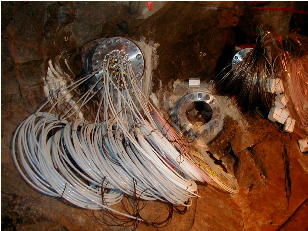
Figure 5-7. Cable package in place.
