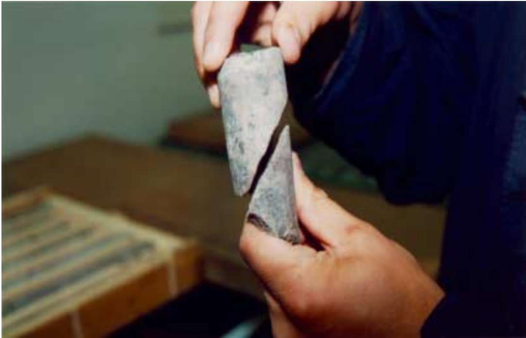
Figure 4-2. The main contributor to the 700 l/min inflow in KA2563A: a single fracture centimetre wide fracture at L=103 m. The structure was subject to extensive grouting, cf Section 2.1.1. The fracture is interpreted as Structure #5 and is interpreted to be closely linked to several sub-parallel structures.
