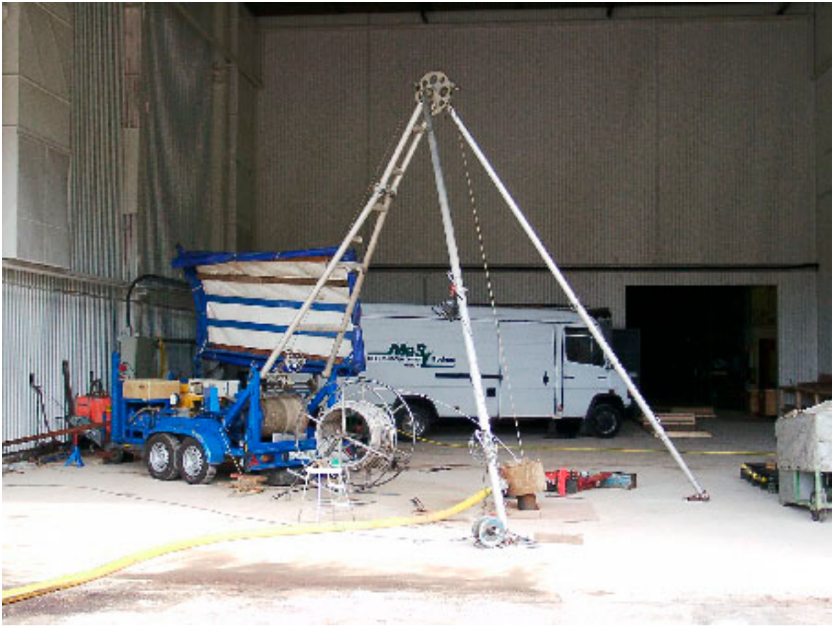
Figure 3-1. Set-up of the MeSy winch MKW 1500 - 20 kN on the top of borehole KOV01 in the SKB store building at Oskarshamn
