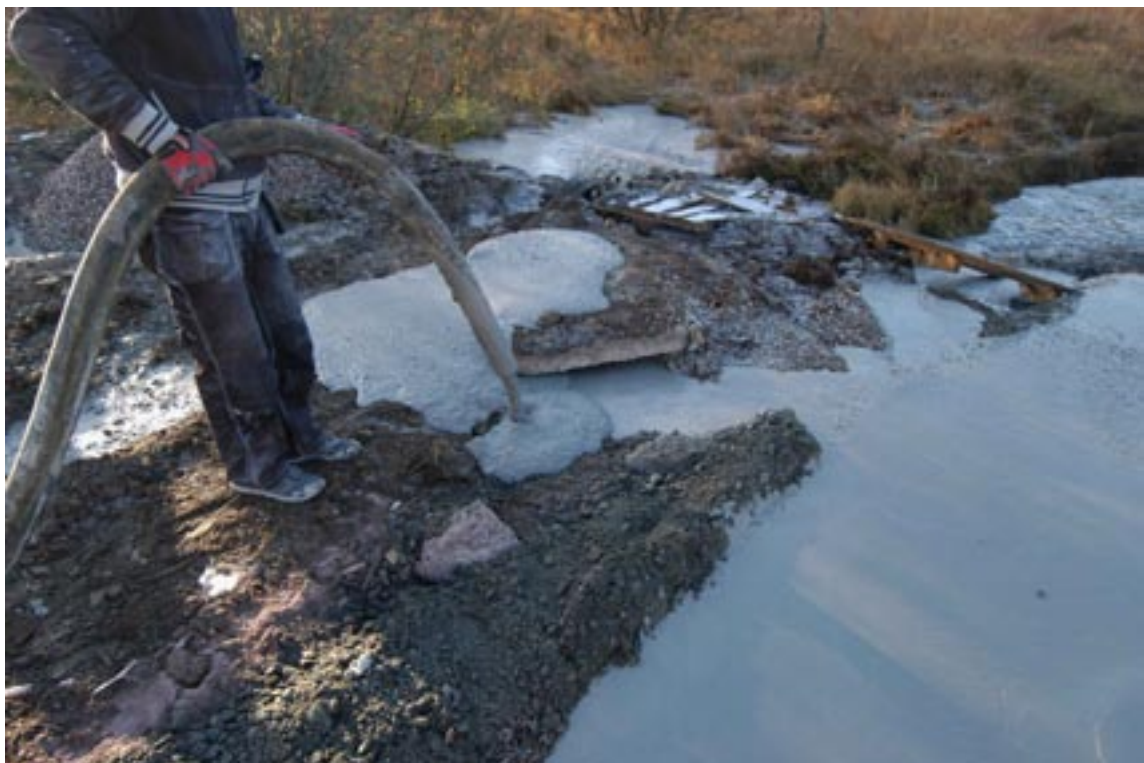
Figure 4-2. Pumping test with small pump and 2.5" hose.
