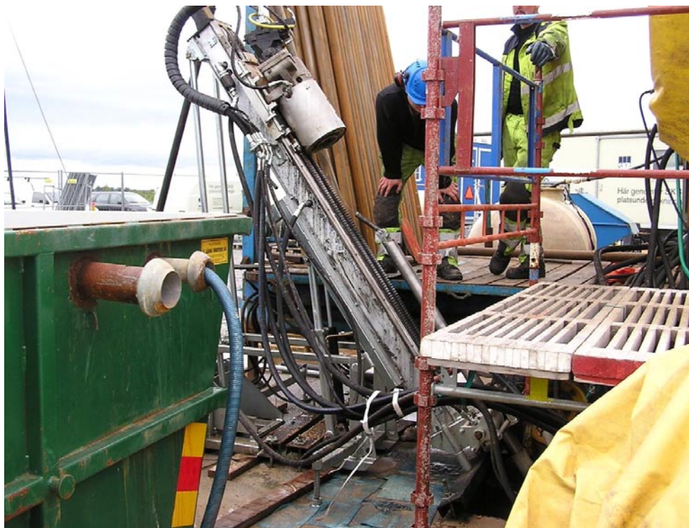
Figure 3-1. The rig Sandvik DE130 cleaned and reamed the borehole KFR27.
