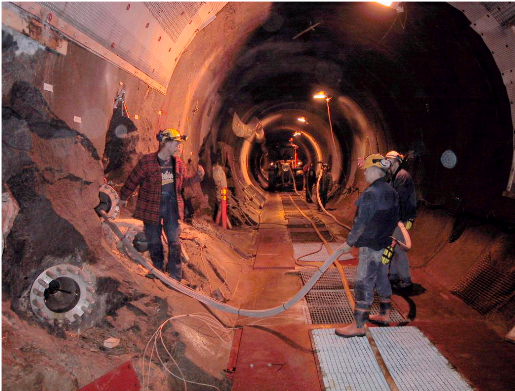
Figure 3-6. Tubes and cables being installed in a lead-through hole.
