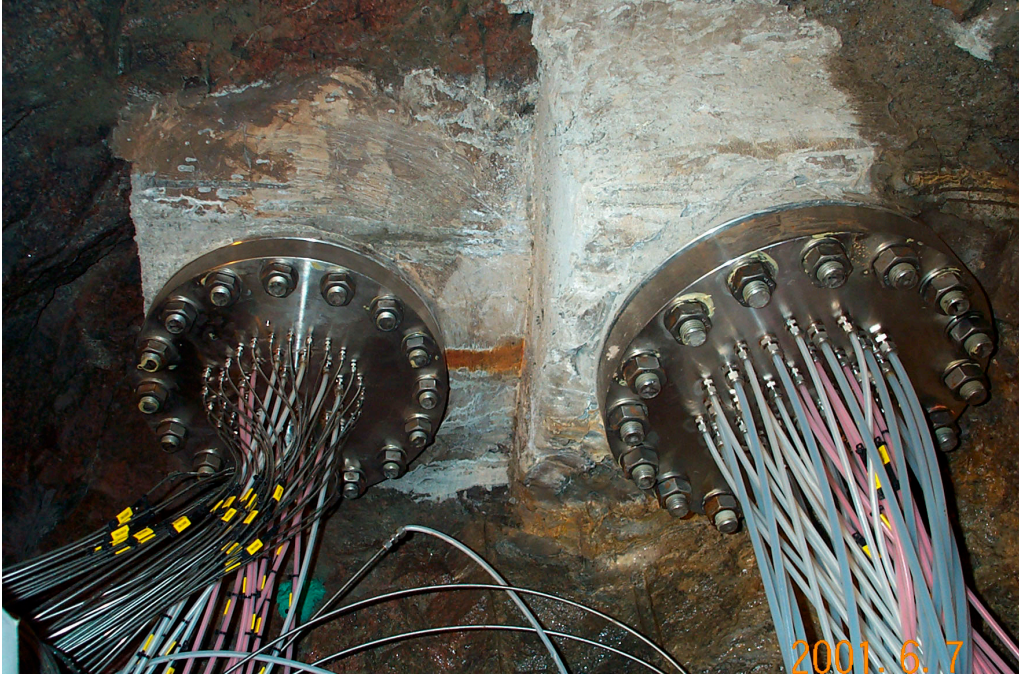
Figure 3-7. Lead-through holes.
