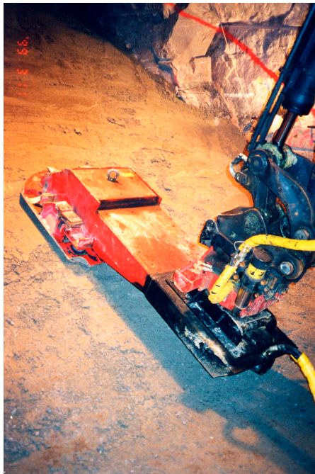
Figure 4-1. Equipment used for compaction.
