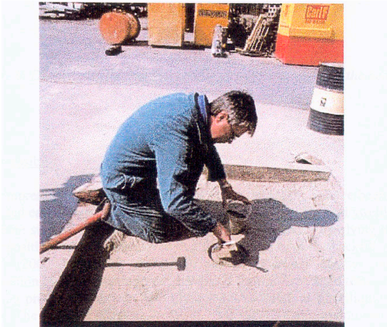
Figure 3-2. Volumeter testing of the density of Friedland clay in earlier compaction test in a 1.5x1.5 m 2 steel frame using a 400 kg vibrating plate [3].
