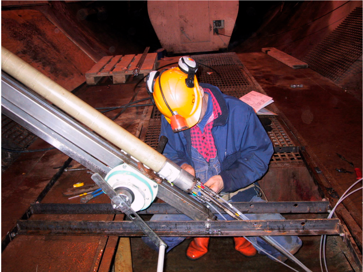
Figure 2-8 Rig for the bentonite packer installation.
