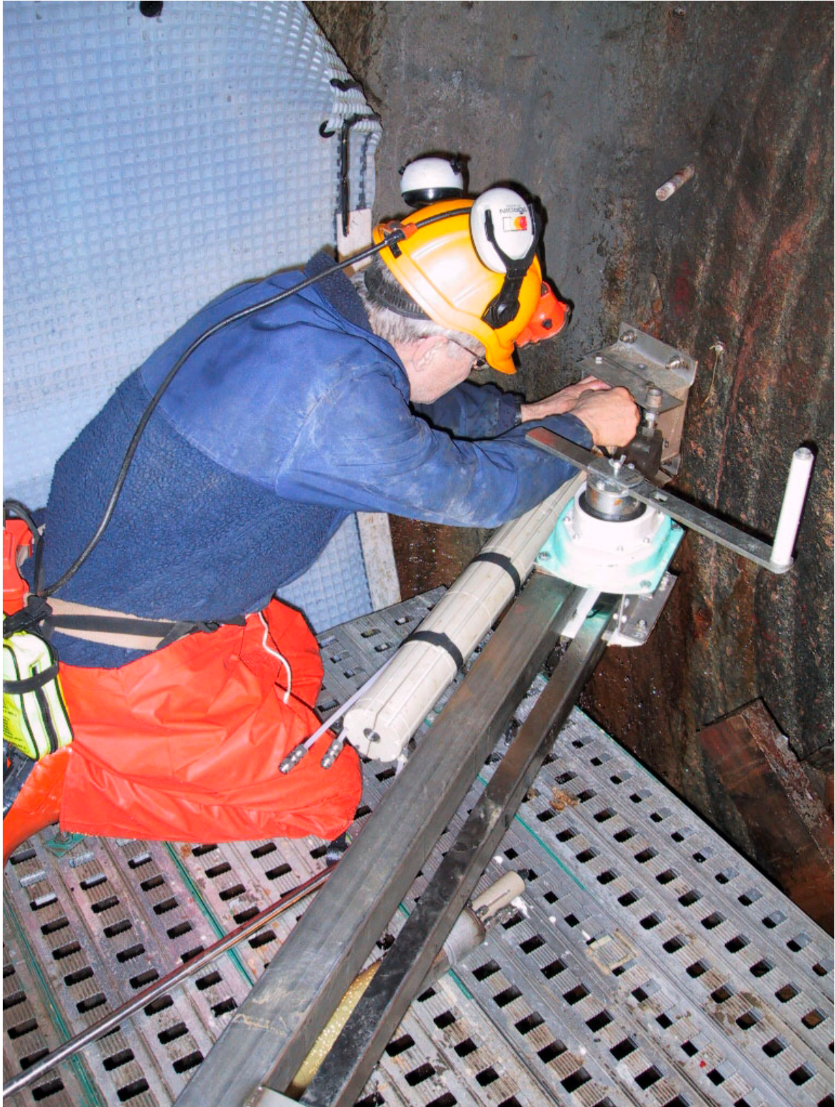
Figure 2-6 Rig for the bentonite packer and the dummy installation.
