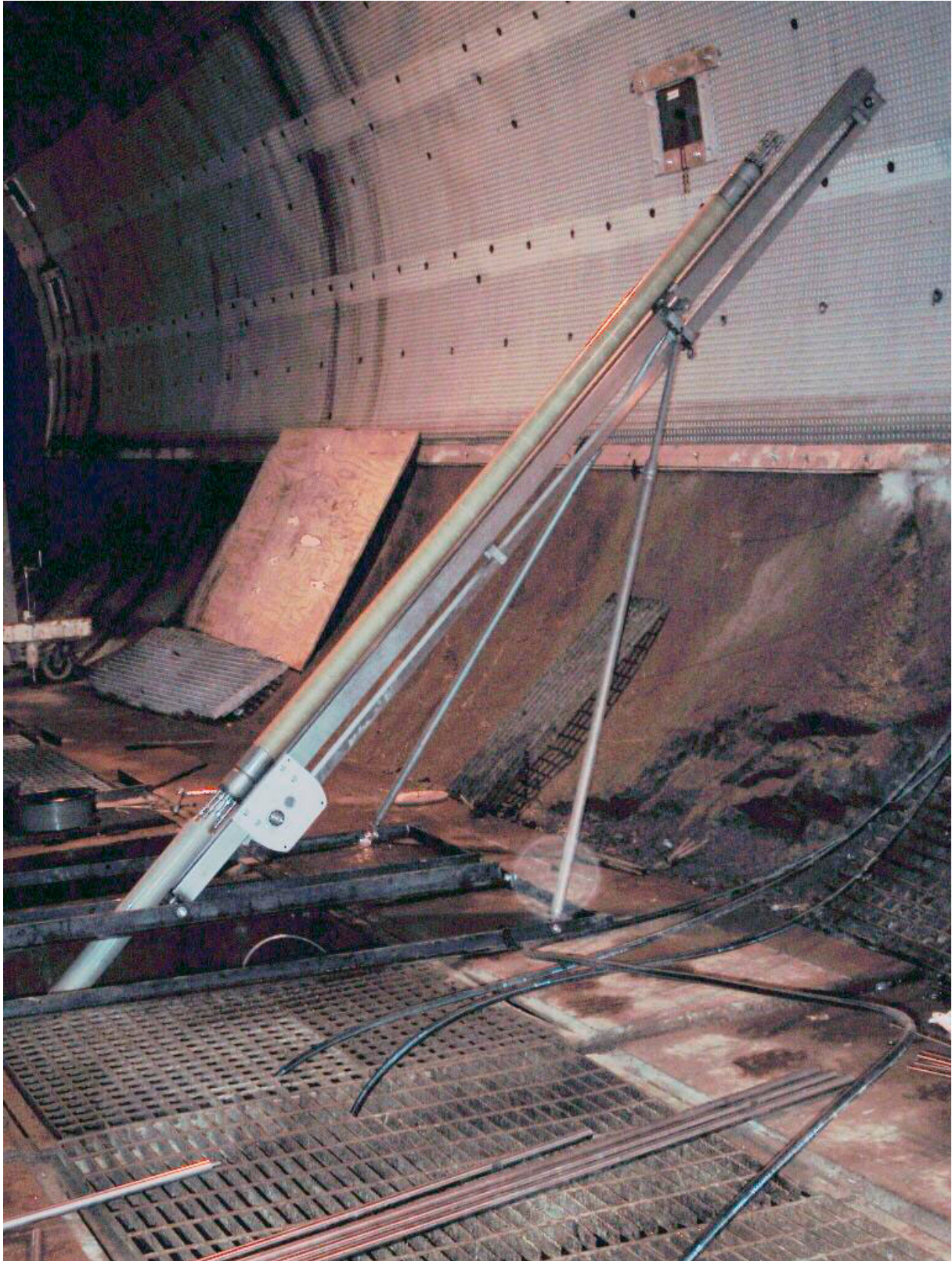
Figure 2-7 Rig for the bentonite packer installation.
