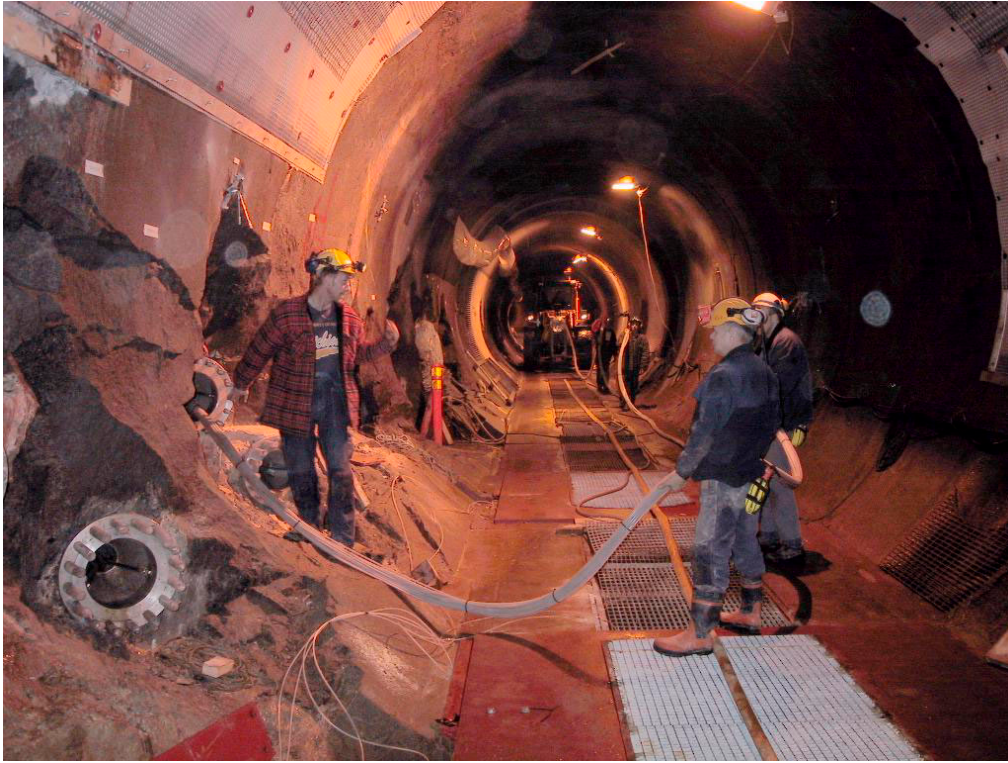
Figure 2-22 Tubes and cables being installed in a lead-through hole.
