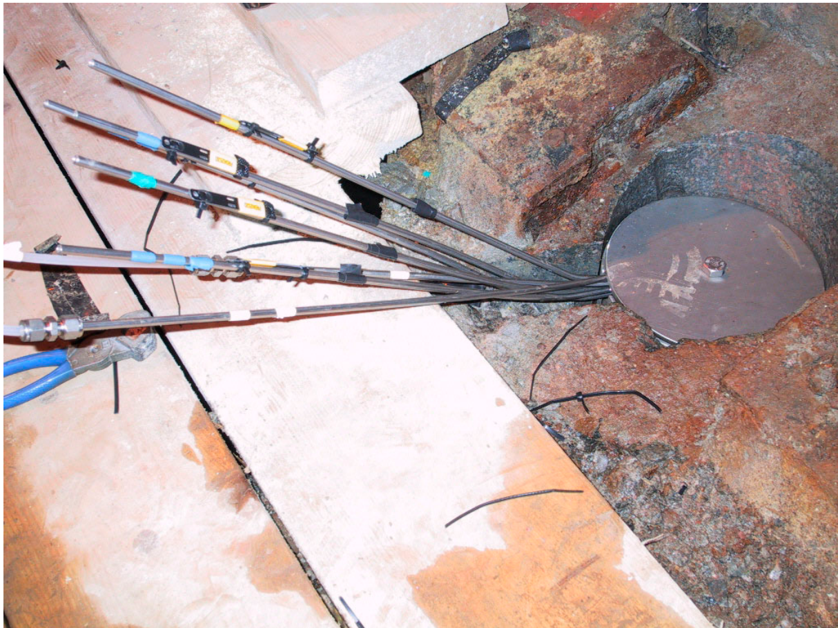
Figure 2-9 Tunnel-floor borehole covered with steel plate.
