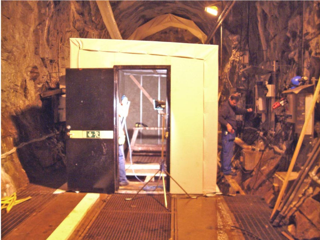
Figure 4-7. Photograph of the insulating construction on top of the experiment volume.
