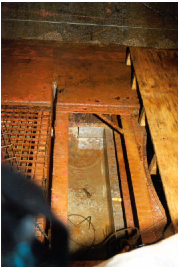
Figure 4-2 One of the weirs closely up-gradient of a deposition hole
