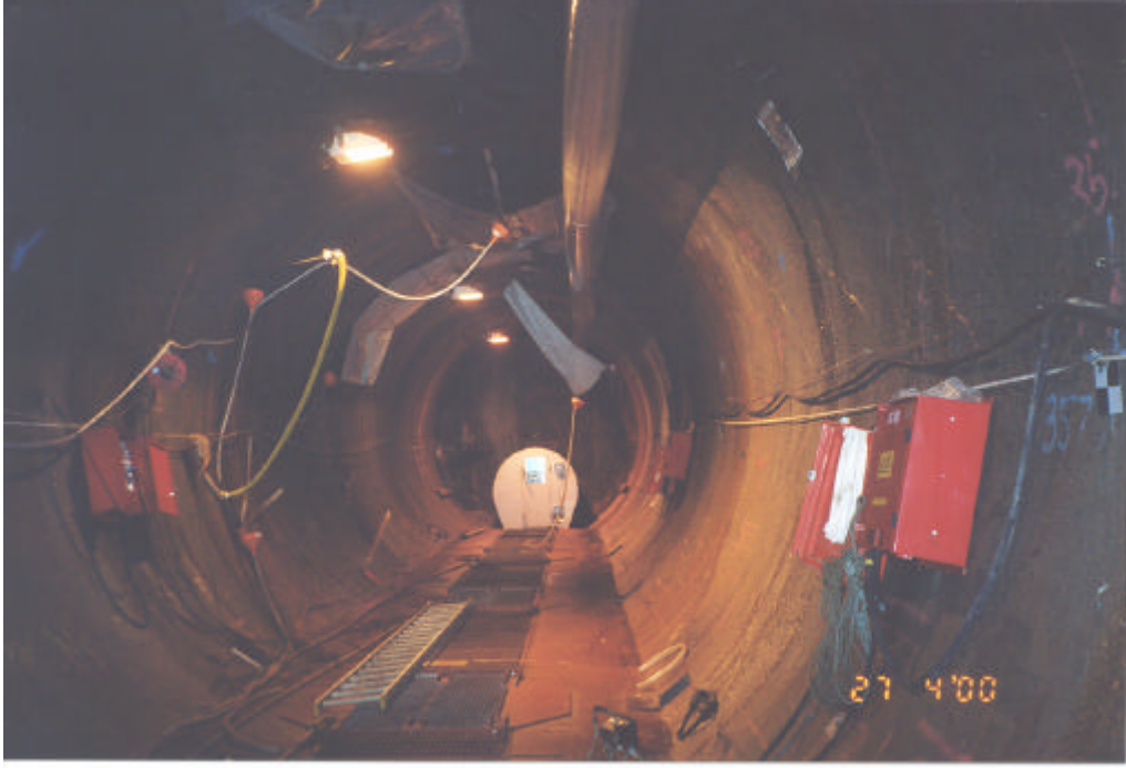
Figure 4-3 The inner section of the prototype repository tunnel
