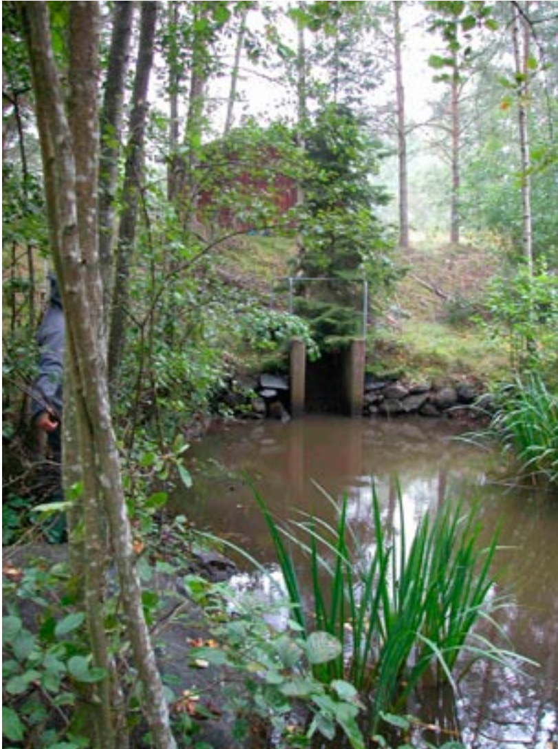
Figure 4-33. Pumping station in the Söråmagasinet reservoir pumping freshwater into the reservoir from Laxemarån.
