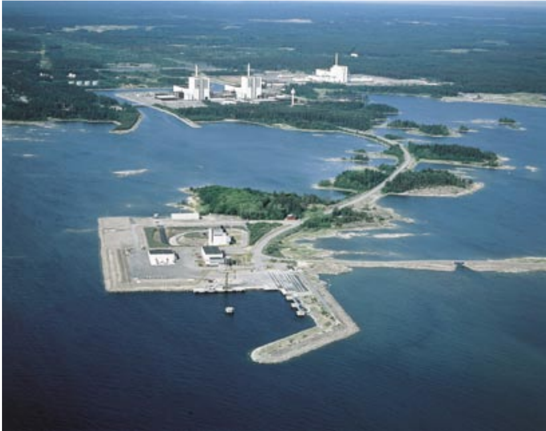
Figure 1-1. Overview of the surface part of the facility at the harbour in Forsmark.
