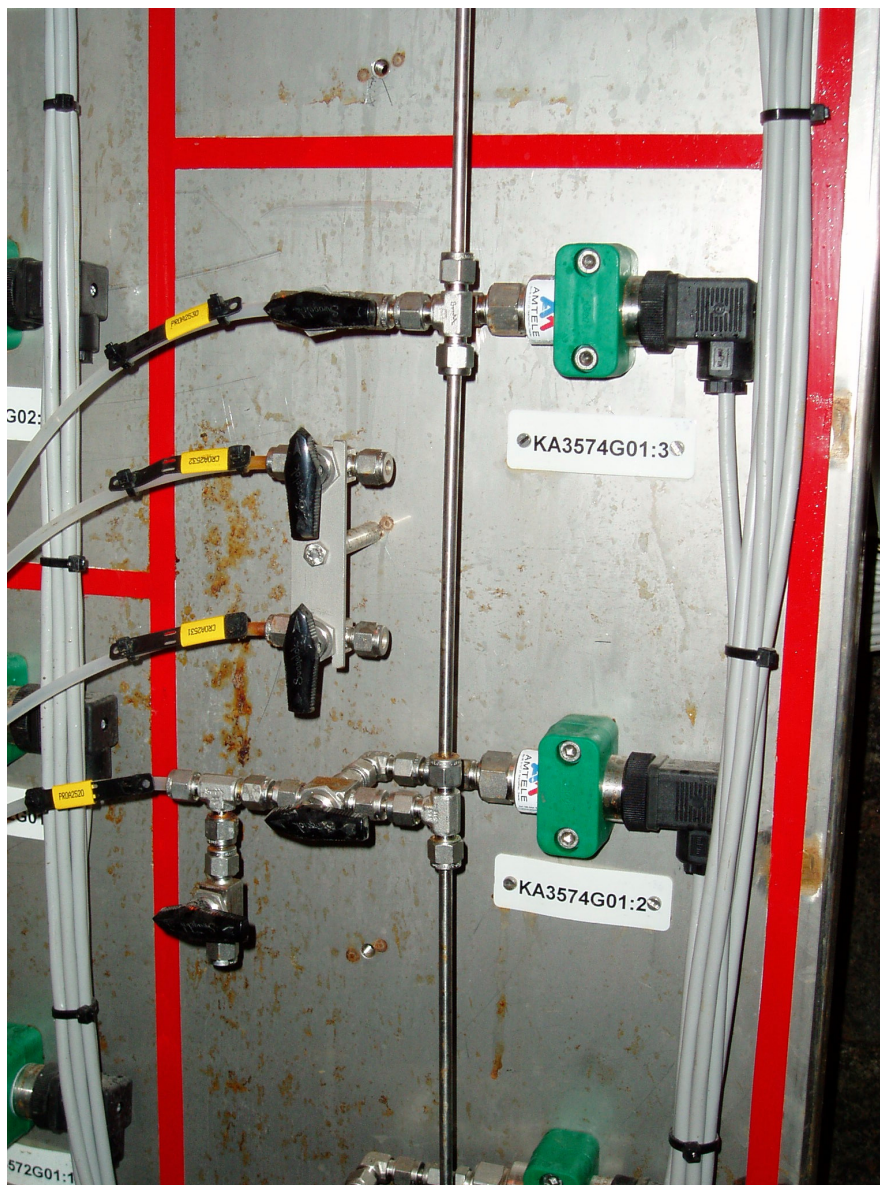
Figure 4-2. Pressure transducers connections.
