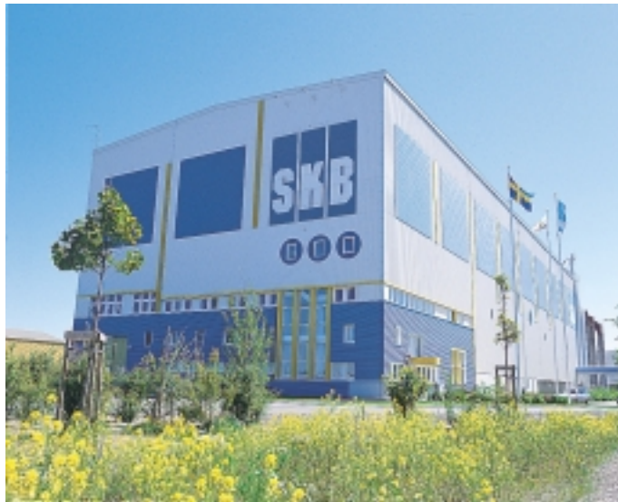
Figure 2-1. Canister Laboratory in Oskarshamn.
