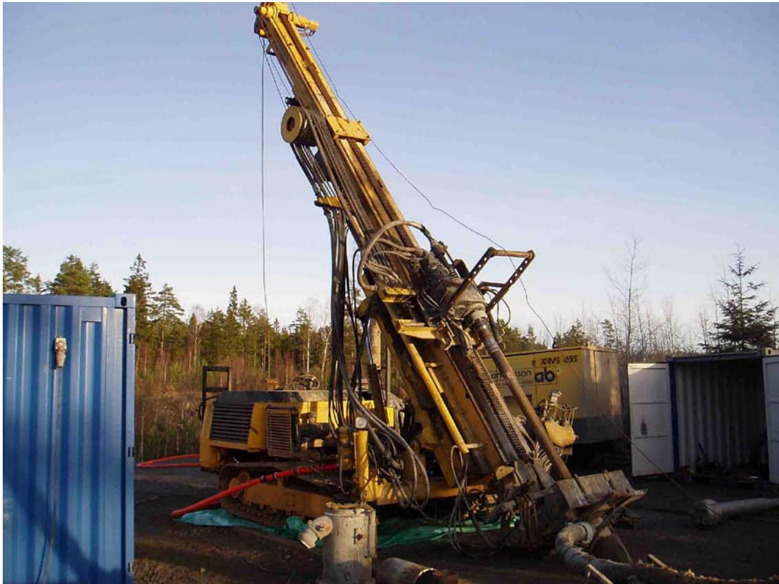
Figure 4-1. The Puntel percussion drill rig at the KLX15A site.
