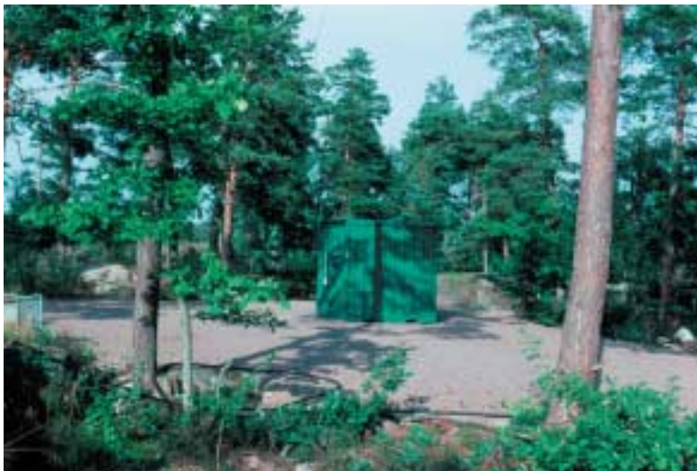
Figure 2-2. Drilling site with measurement container placed over a finished borehole, in this case with equipment for long-term monitoring of groundwater levels.
