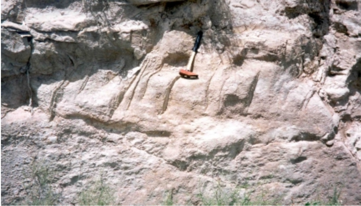
Figure 2-3. En echelon pinnate joints with vein fill, on a fracture face. Suggests sinistral strike slip movement on fracture (fault?) face. Road cutting west of Maqarin station.
