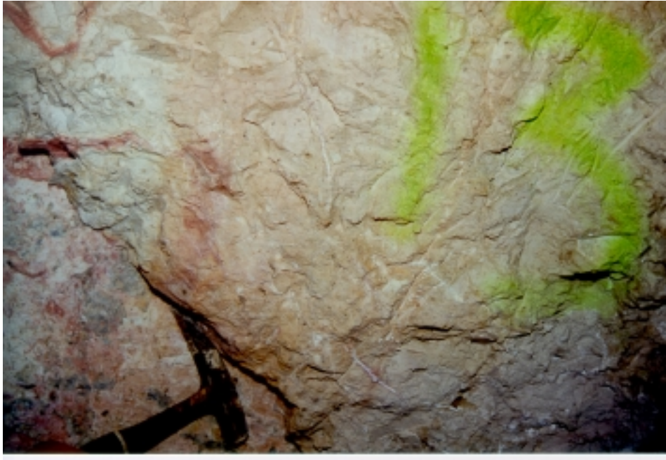
Figure 3-4. Transition zone profile; Sample location TZ (+3b). Transition between cement-like material (white and red, left) and strongly baked marl (brown to grey, right) is clearly visible.
