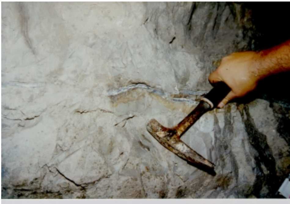
Figure 3-3. Transition zone profile: Sample location TZ(-1); adit roof fracture.
