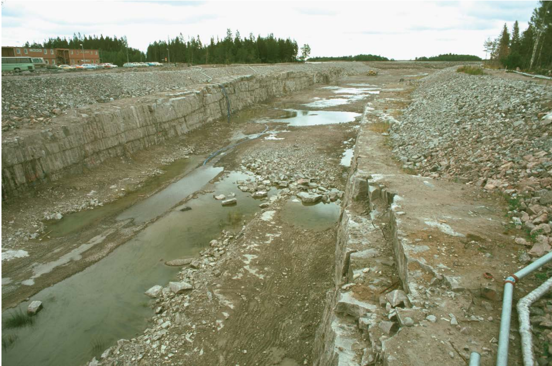
Figure 3-22. Picture from the construction of the 13 m deep and more than one kilometre long canal between the Baltic Sea and the nuclear power reactors. Horizontal fractures/sheet joints are encountered along the entire excavation. There are several “horizons” of extensive sheet joints on top of each other. The picture is taken from the southern side of the canal where the bridge crosses the canal between drill sites 7 and 8, see Figure B-1 in Appendix B.
