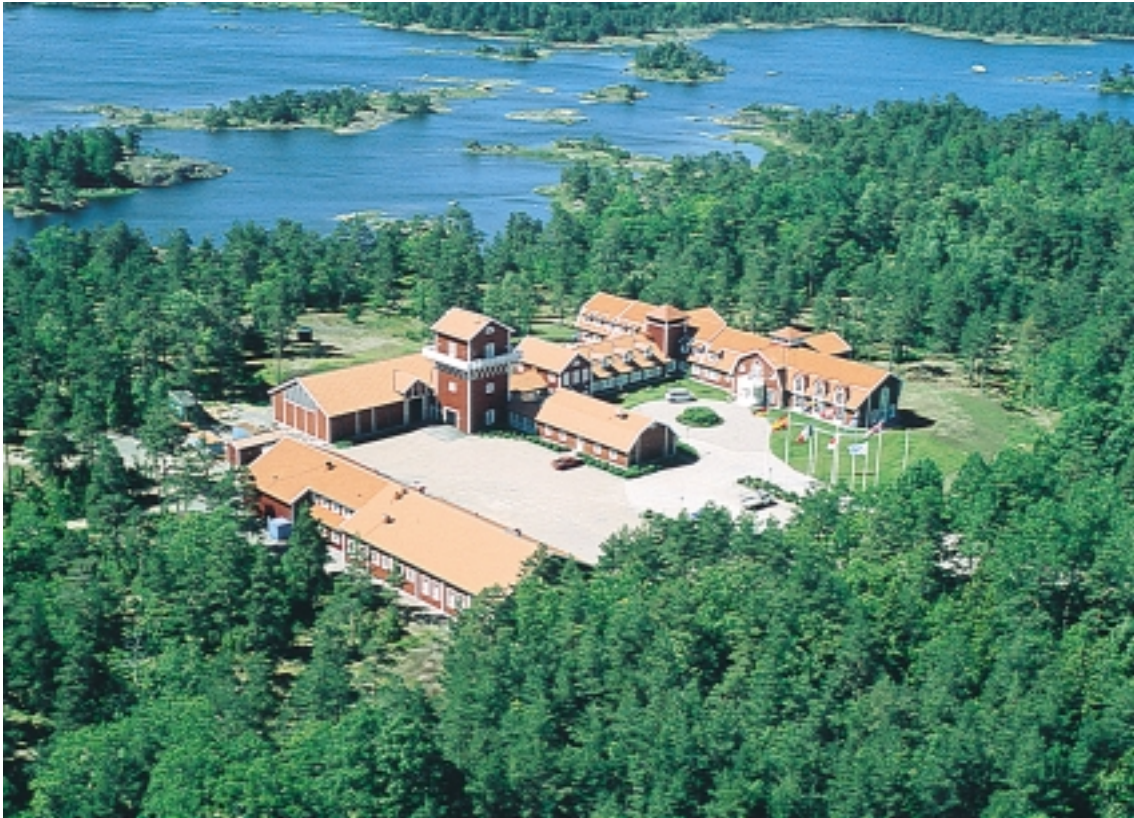
Figure 1-3. Overview of the Äspö Research Village.
