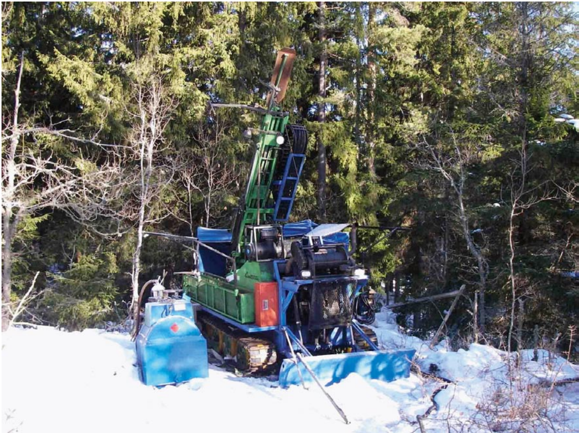
Figure 3-1. The Geomachines GM200 drill rig.
