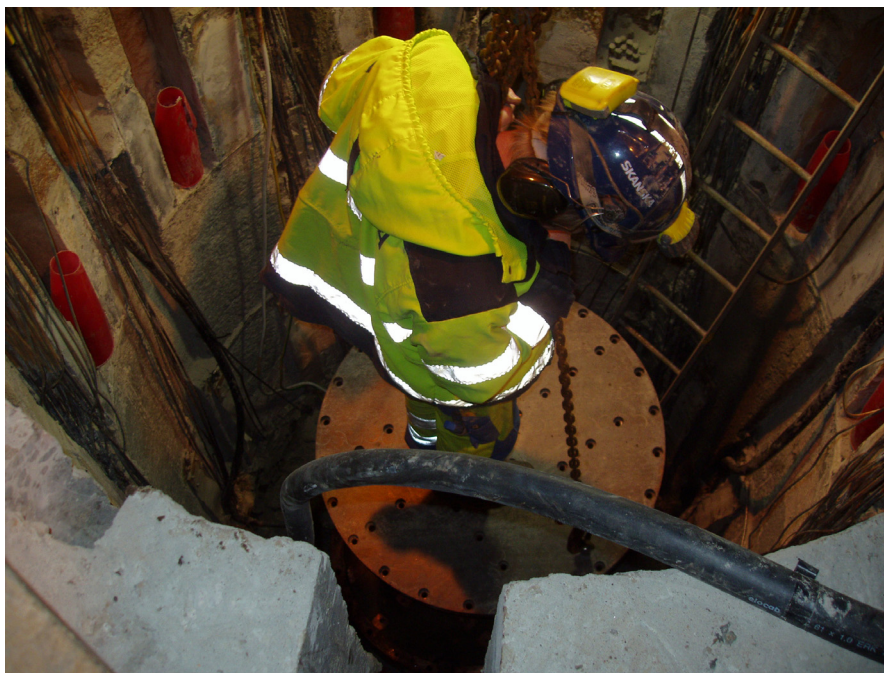
Figure 6-1. The upper lid is lifted up from the deposition hole.
