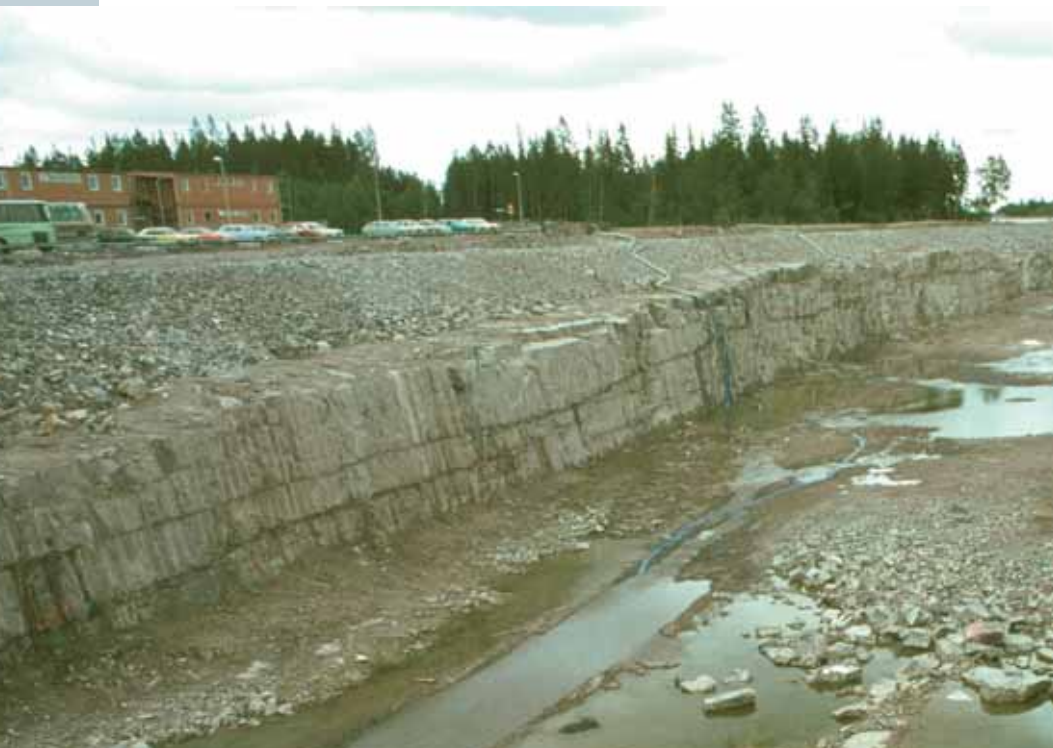
This is what it looked like when the cooling water channel to the nuclear power reactors was blasted in the 1970s. In the channel wall you can clearly see the long horizontal fractures that are so typical of the upper part of the rock in Forsmark.
