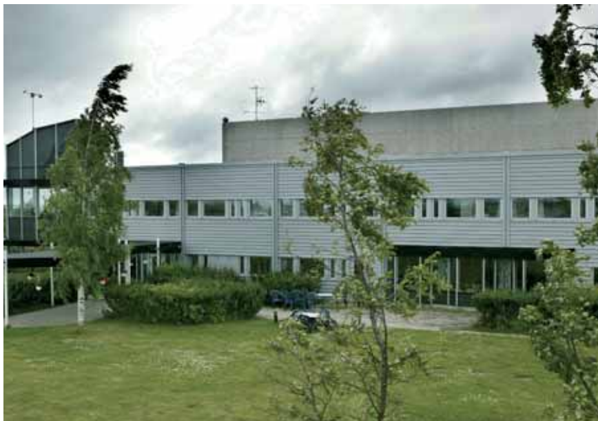
SFR and SKB's site office in Forsmark Harbour.
