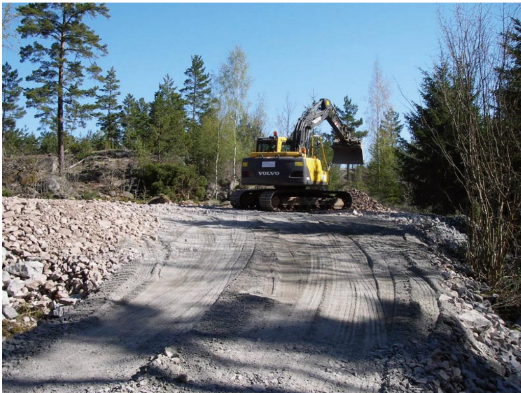
Figure 5-2. Constructing the drill site for borehole KLX19A.
