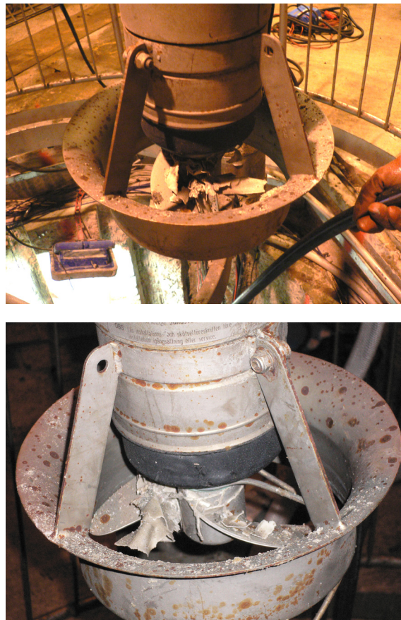
Image 6-1. Mixer with foreign objects in propeller. (Photo: Bo Nirvin, SKB).
