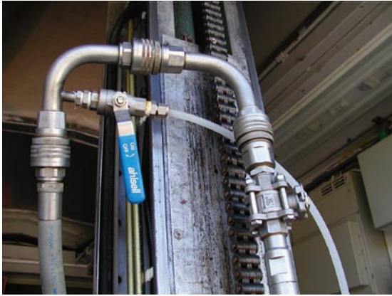
Photo 7. Top of test string with shunt valve and nylon line down to the pump basket.
