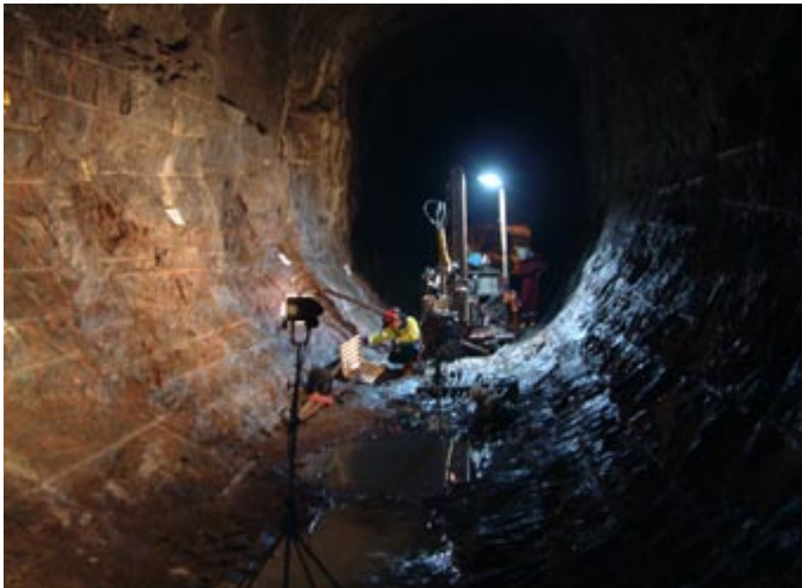
Figure 2-7. The Apse experimental drift shortly after the excavation.
