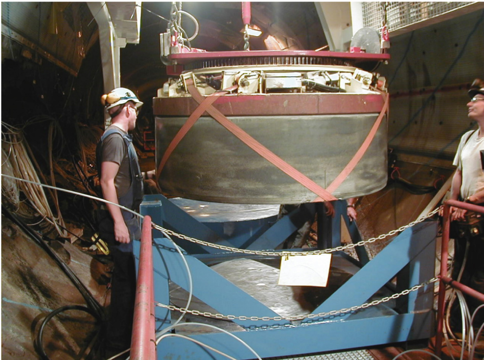
Figure 2-1 Handling of full size bentonite blocks in Äspö HRL.
