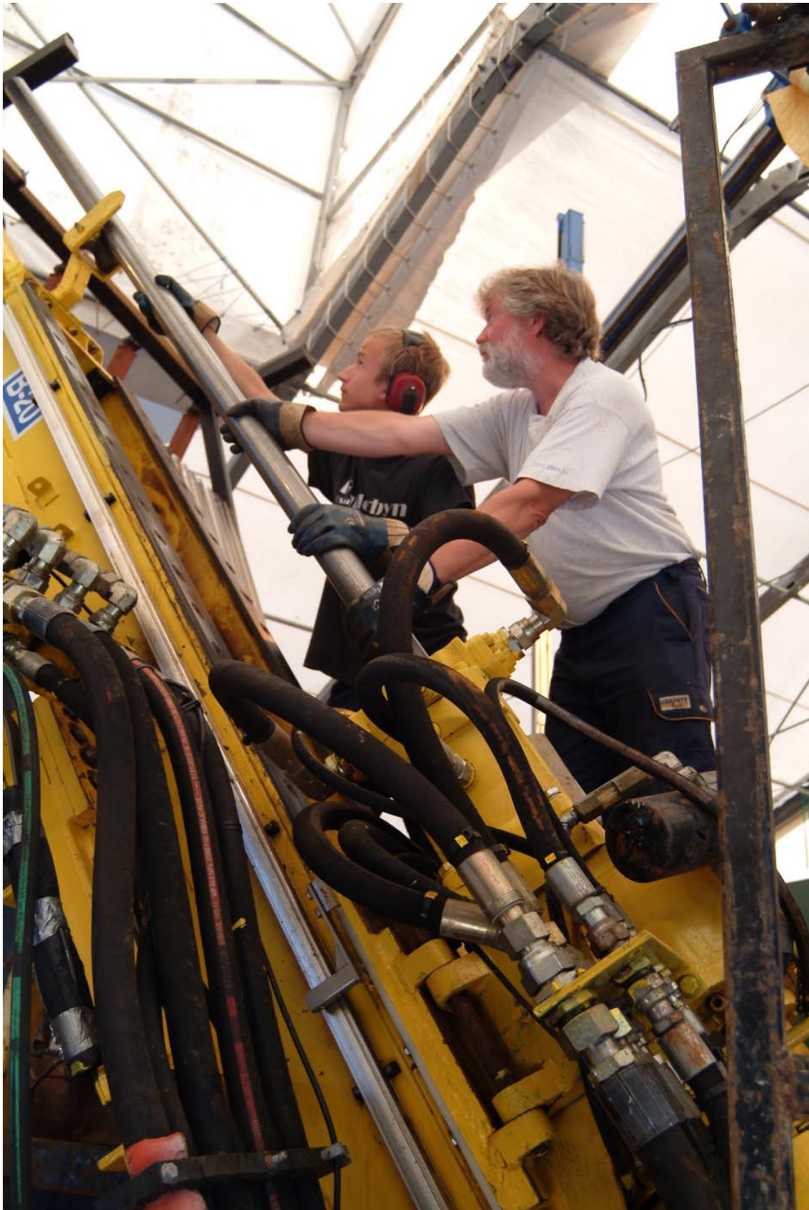
Figure 3-2. The B20 core drilling machine in operation on borehole KFM07B.
