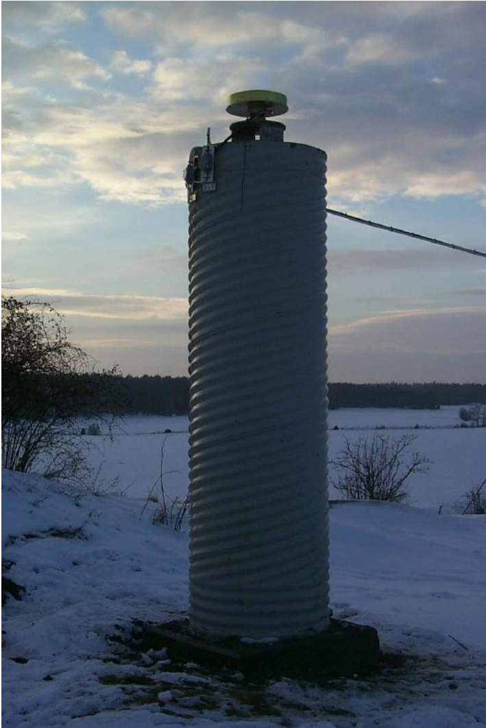
Figure 4-1. The Swepos reference station in Uppsala.
