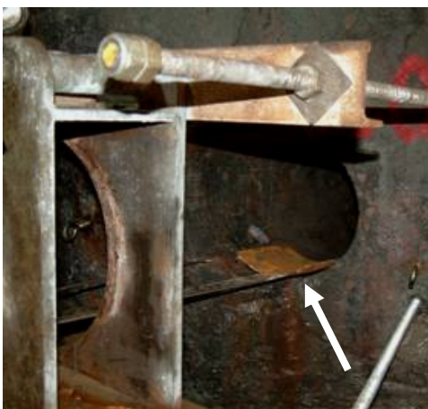
Figure 2-3. Insertion of tool for core breakage.
