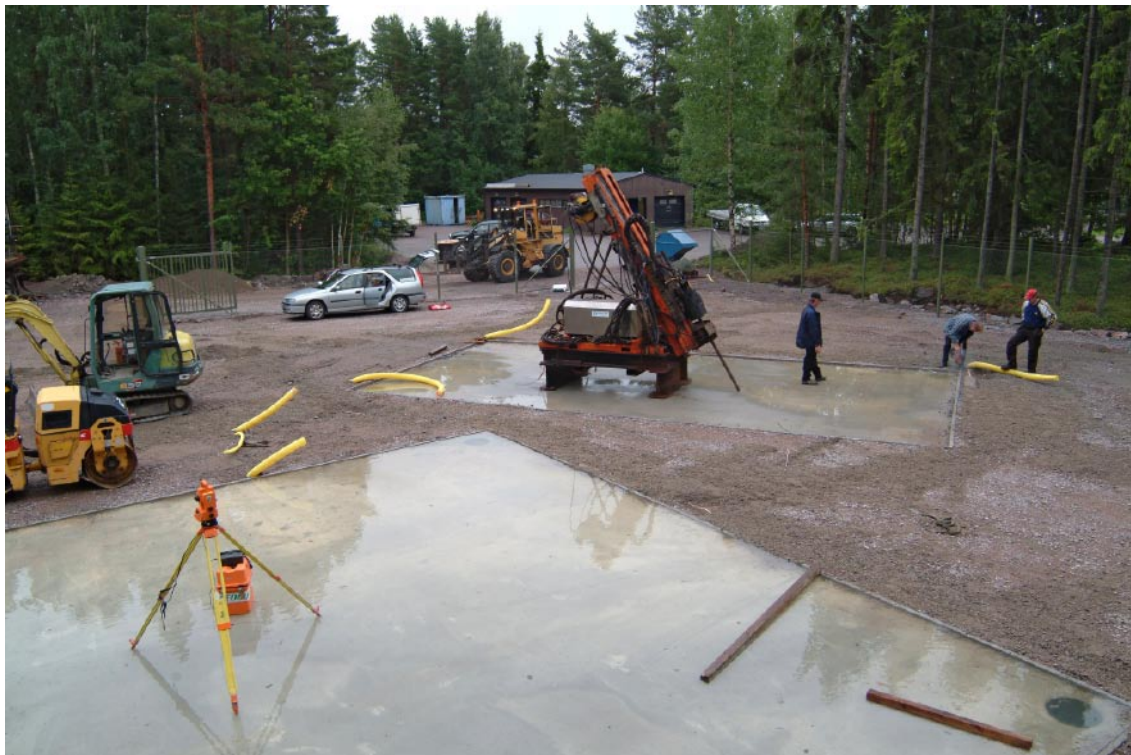
Figure 3-1. The Onram 2000 CCD core drilling machine in operation on borehole KFM09A.
