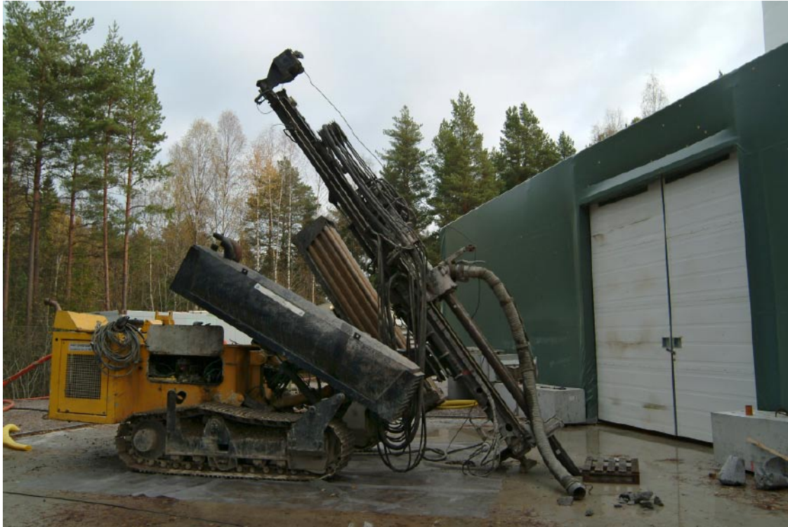
Figure 3-2. Soil drilling with a Nemek 711 percussion drilling machine at borehole KFM09B.
