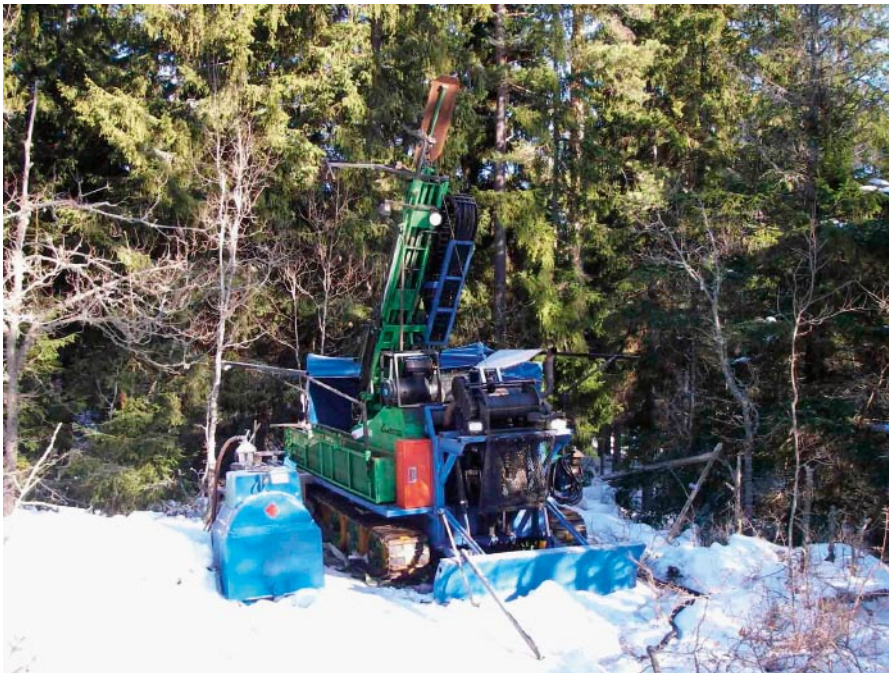
Figure 3-1. The Geomachines GM200 drill rig at KLX10C.
