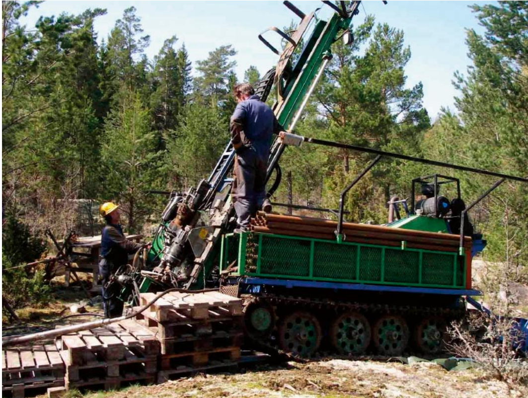
Figure 4-5. Drilling at KLX22A.
