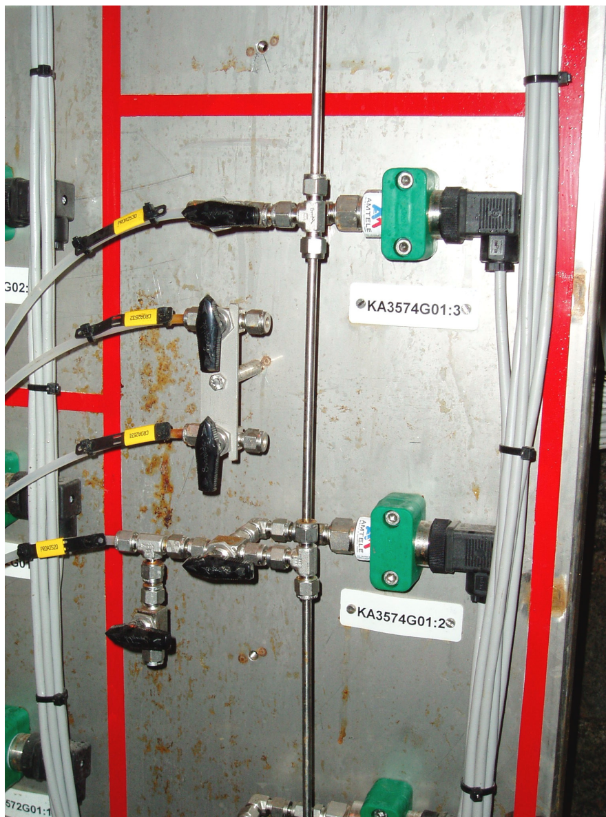
Figure 4-2. Pressure transducers connections.
