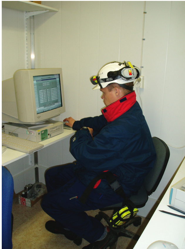
Figure 4-1. All pressure transducers are connected to the HMS system. In the G-tunnel there is a computer in the HMS system where logging frequencies easily can be changed.
