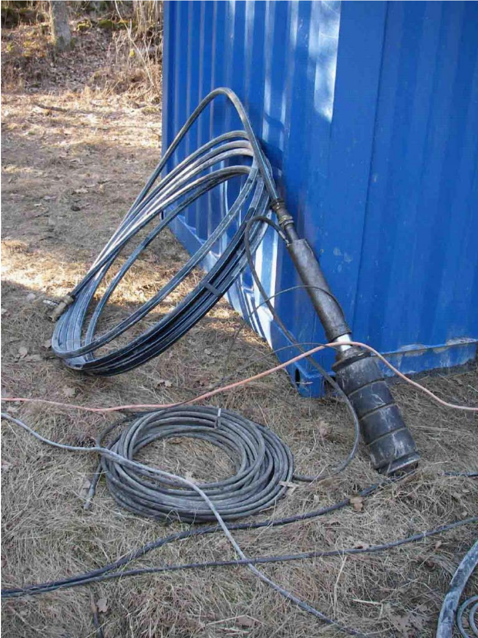
Figure 4-4. Tremie pipe and packer for casing grouting.
