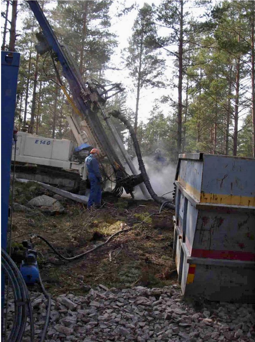
Figure 3-1. Drill site HLX40 with the Enteco E14G drill rig.
