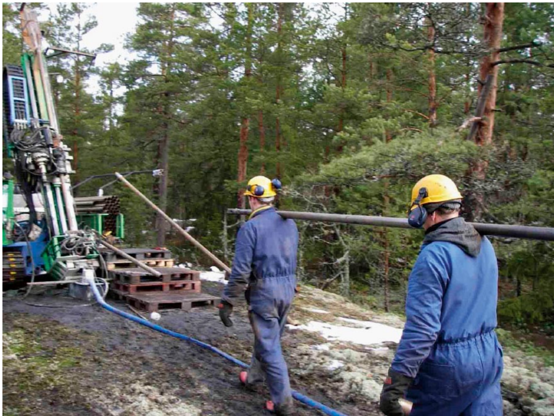
Figure 4-3. Drillers carrying the core barrel at the site for KLX11C.
