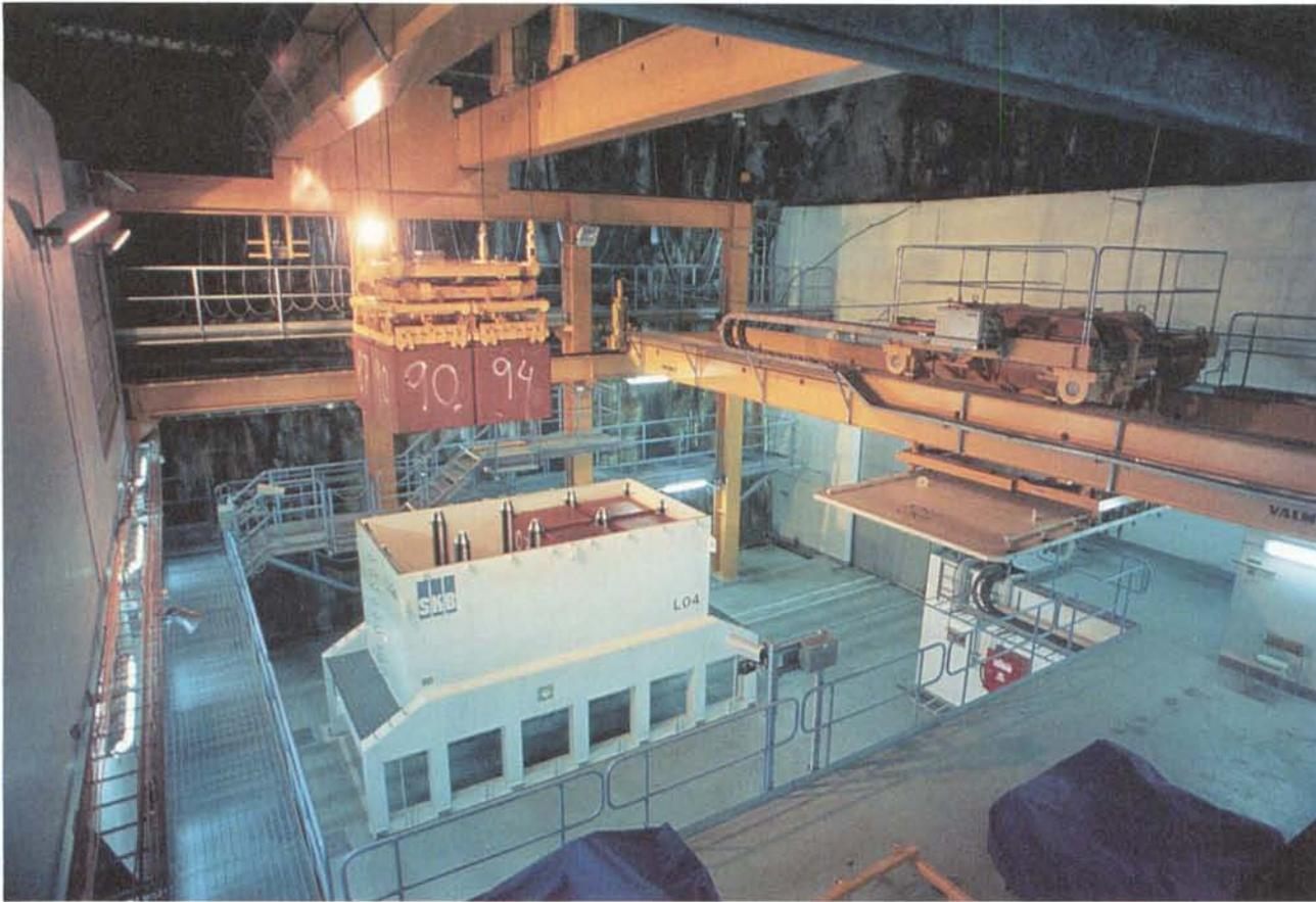
**Figure 4-2.** The operational waste is transported in special transport containers. In SFR the waste packages are unloaded with remote-controlled handling equipment.
