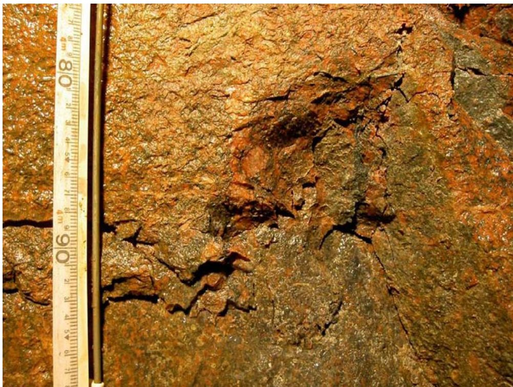
Figure 11. The anticipated location of a sample MD at the depth of 4,90m. Strong oxidation can be seen in the picture.
