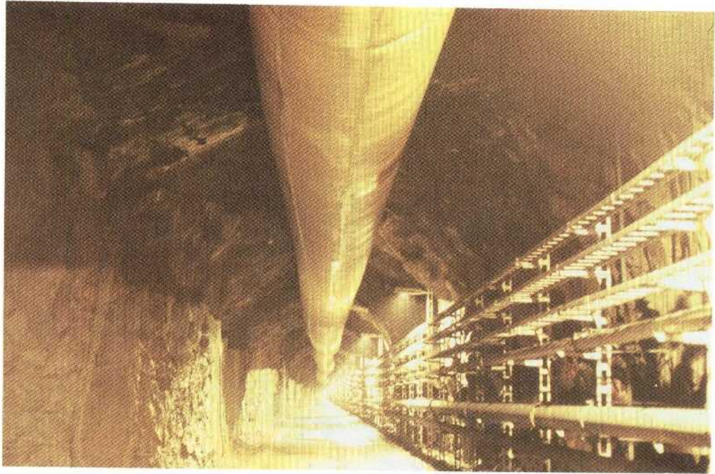
Figure 4.7 The Äspö access tunnel from 205 m and downwards. The height and width are 5.5 m x 5.5 m respectively and the inclination is 7 %. The large tube under the tunnel roof is the ventilation. The picture was taken the 17 of August 1993.
