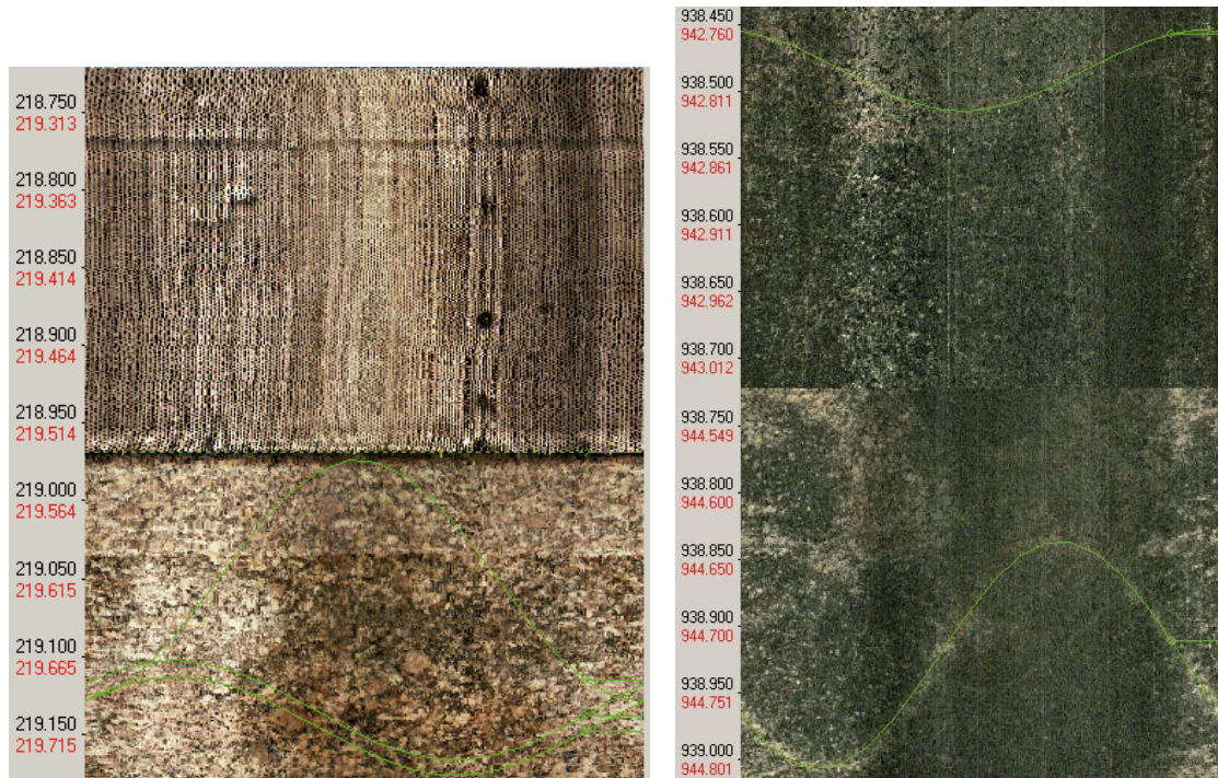
Figure 4-1. Left – Picture of metal sheet placed in the KLX08 borehole. Right – Picture that shows the missing BIPS-image in KLX08. Notice the change from dark grey/black borehole wall to a brighter and diffuse image in the middle of the picture. The two green lines that marks two mapped features are actually c 2 m apart.
