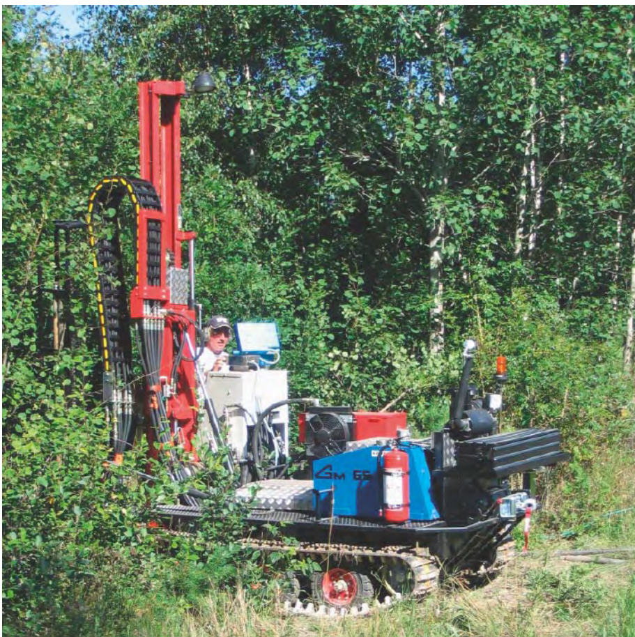
Figure 3-42. Soil drill rig.
