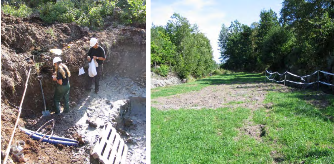
Figure B-2. Trench for Quaternary deposit mapping before and after remediation.
