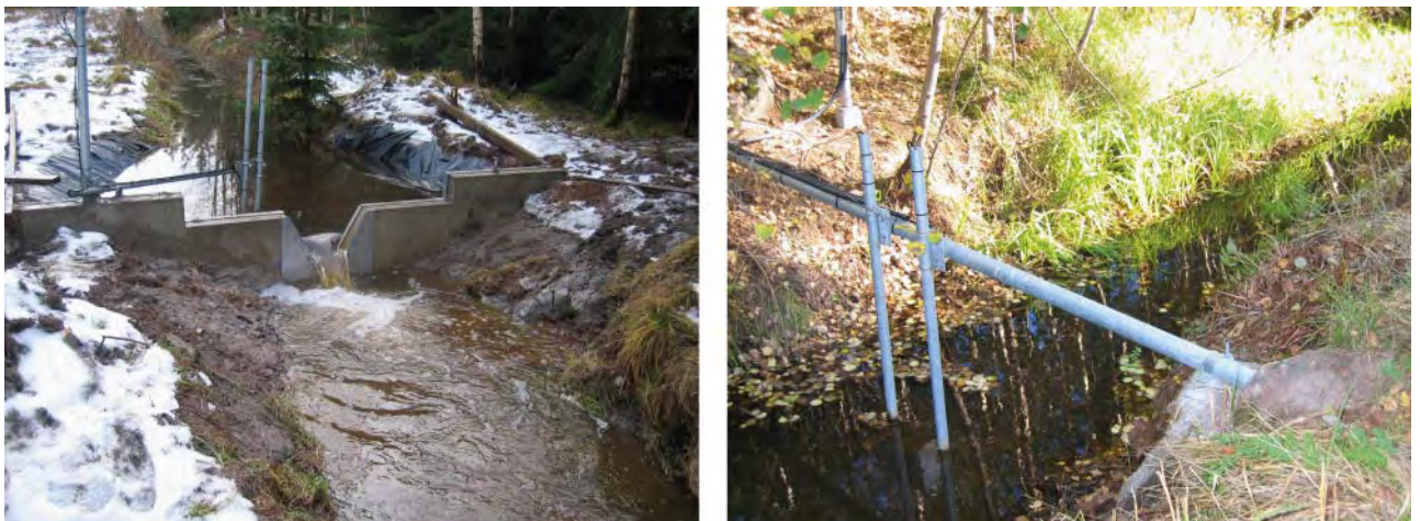
Figure 3-45. Stream discharge stations. The left-hand picture shows the weir at monitoring station PSM000347. The right-hand picture shows monitoring station PSM000353 at a naturally constricting section. The locations of the stations are shown in Figure 3-46 below. Sensors for measurement of level, temperature and electrical conductivity are mounted on poles in the middle of the stream.
