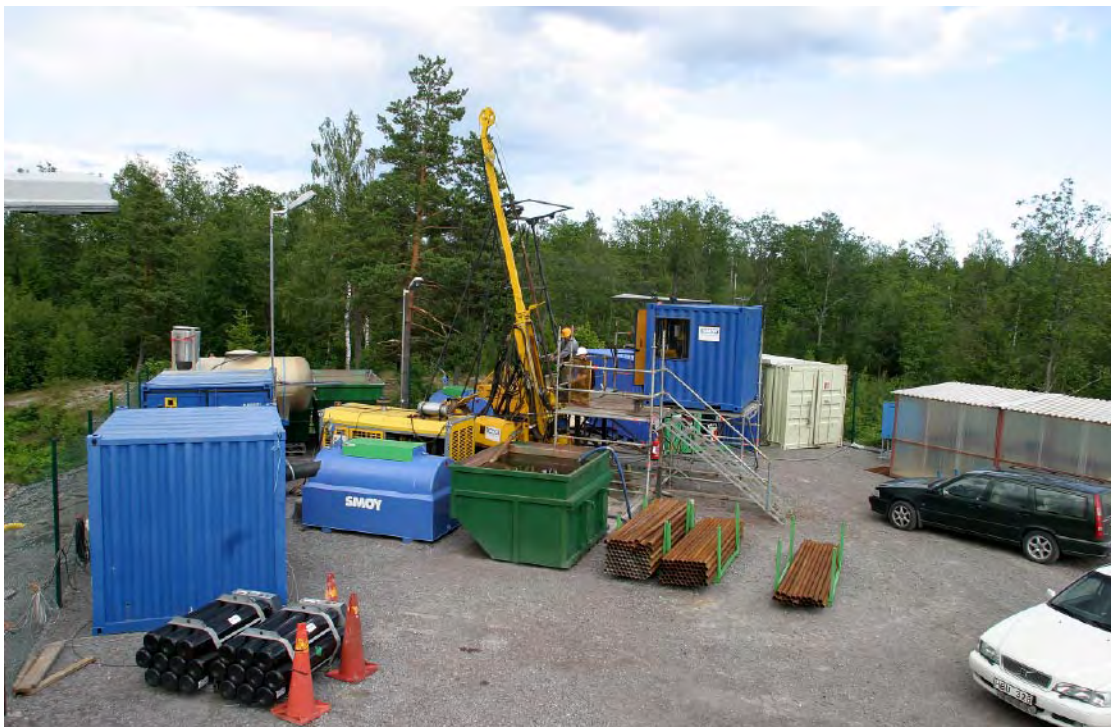
Figure B-3. Drilling site KLX03 in the Laxemar subarea.
